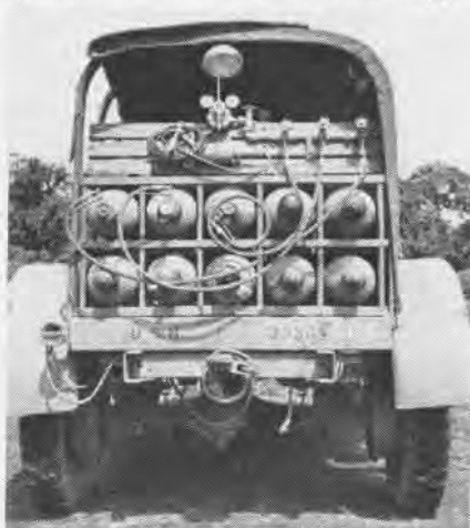
OXYGEN TRUCK HOLDS COMPLETE REPAIR SHOP
