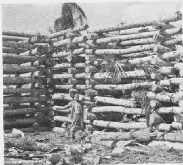
Log revetment for aircraft being constructed by the Japanese when Marines invaded Betio Island, shows typical building technique
