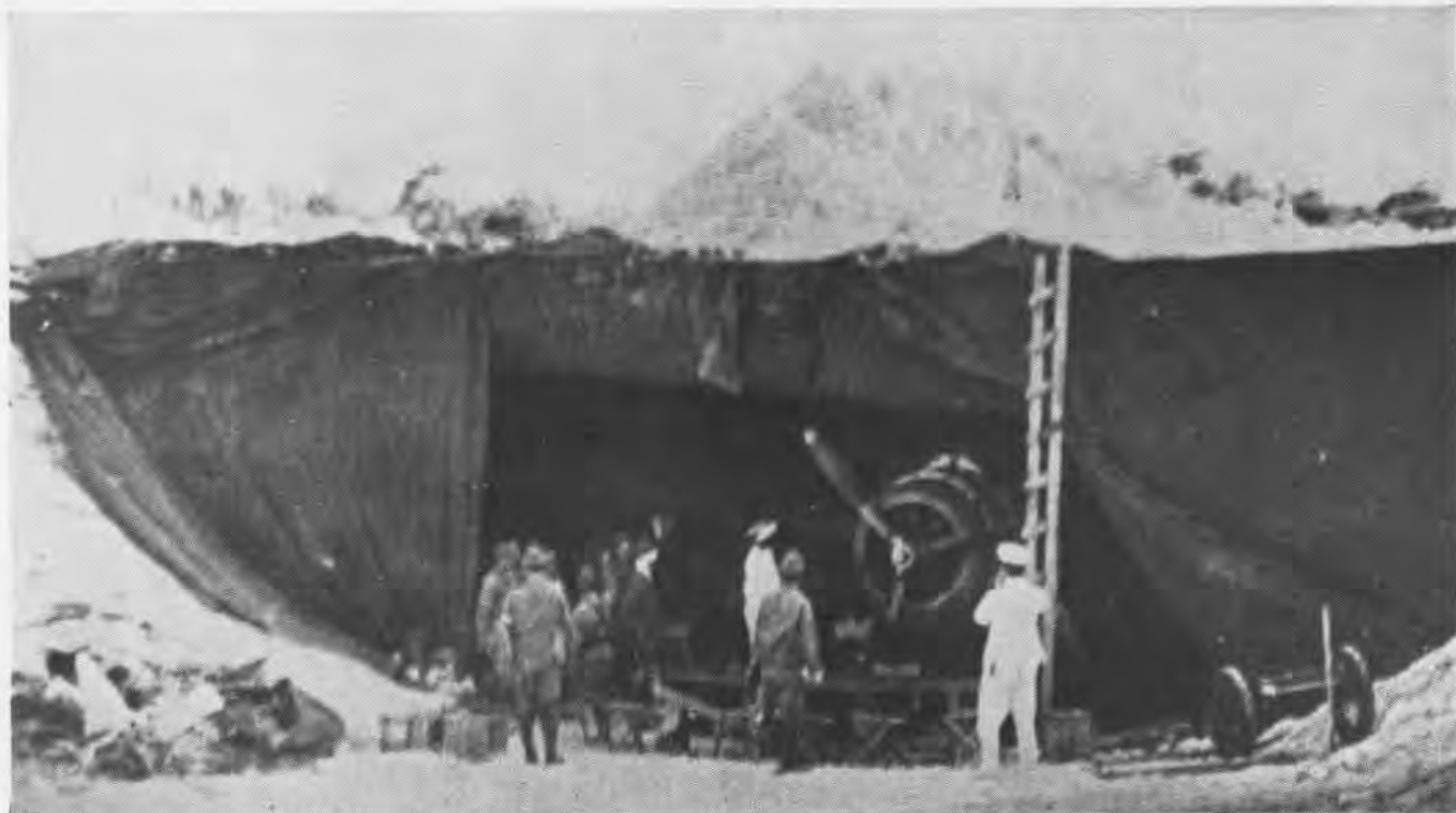
CAPTURED PHOTO SHOWS JAPS INSPECTING UNDERGROUND PLANE HIDE AT EDGE OF MARINE AIR STRIP ON WAKE ISLAND. CURTAIN CONCEALS PLANE
