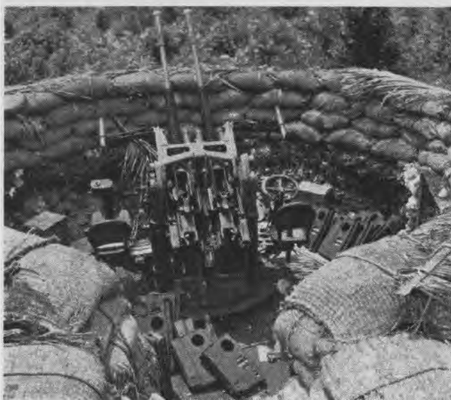
Straw sand bags reinforce revetment of this 25 mm. AA gun at edge of Agana airfield. Shell clips rest in framed enclosure, right
