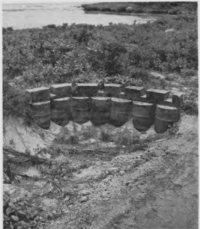
CONCRETE GUN CREPELLATION RESTS ON DRUMS IN ROADSIDE POSITION
