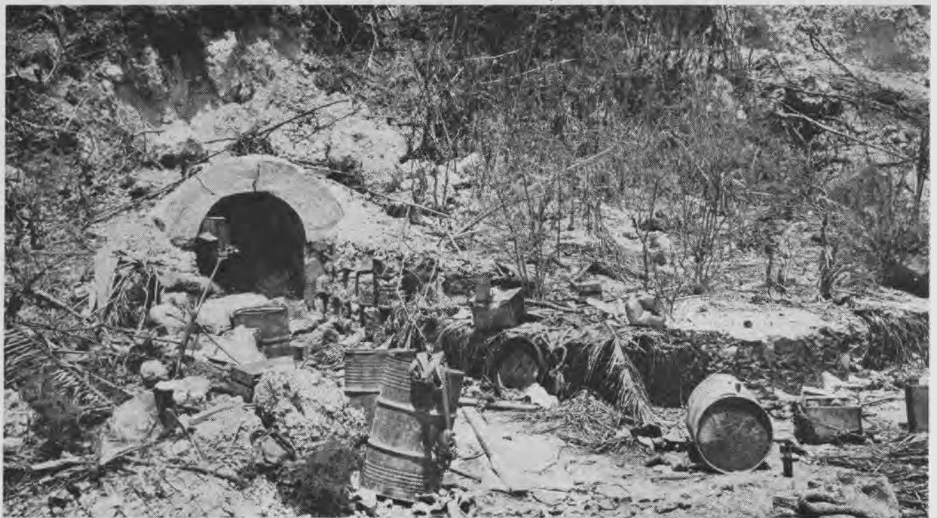
ENTRANCE TO CAVES FOR JAP SUPPLY STORAGE IS MARKED BY CONCRETE-LINED TUNNEL AT FOOT OF GUAM HILLSIDE. VITAL STORES WERE INSIDE
