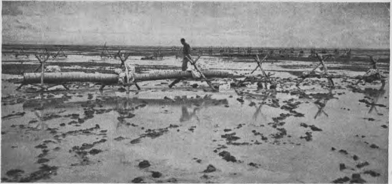
Boat obstacles at Ylig Bay, Guam, photographed at low tide, show the varied use to which the Japs put local materials to build bar-
