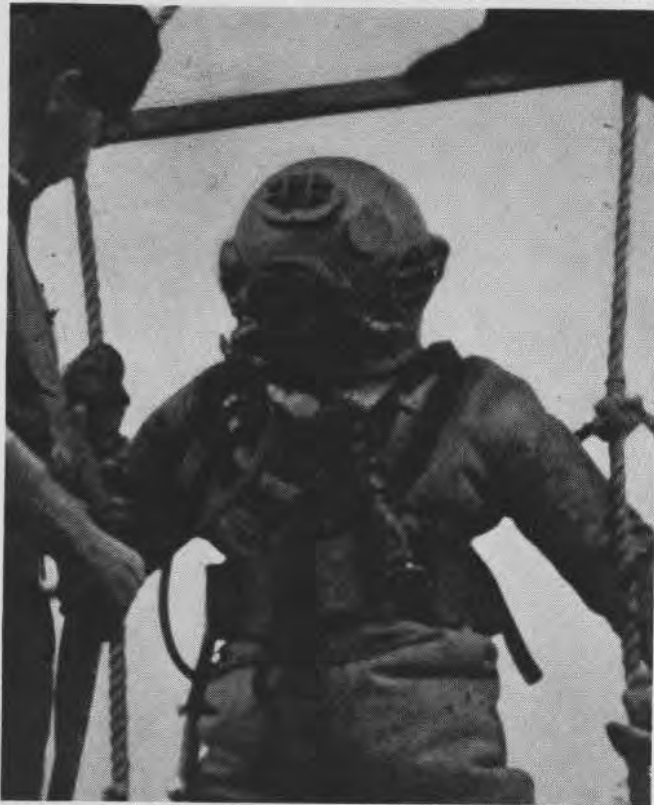
VOLUNTEERING TO FACE A BLAST, NAVAL OFFICER IS LOWERED INTO SEA
