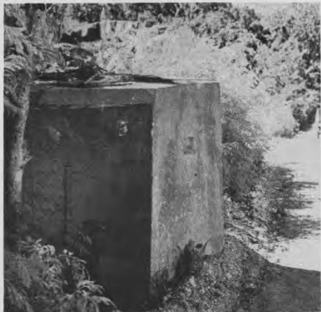
Concrete strong point at roadside has open slots for firing against troops on the road. Concrete is reinforced to protect snipers
