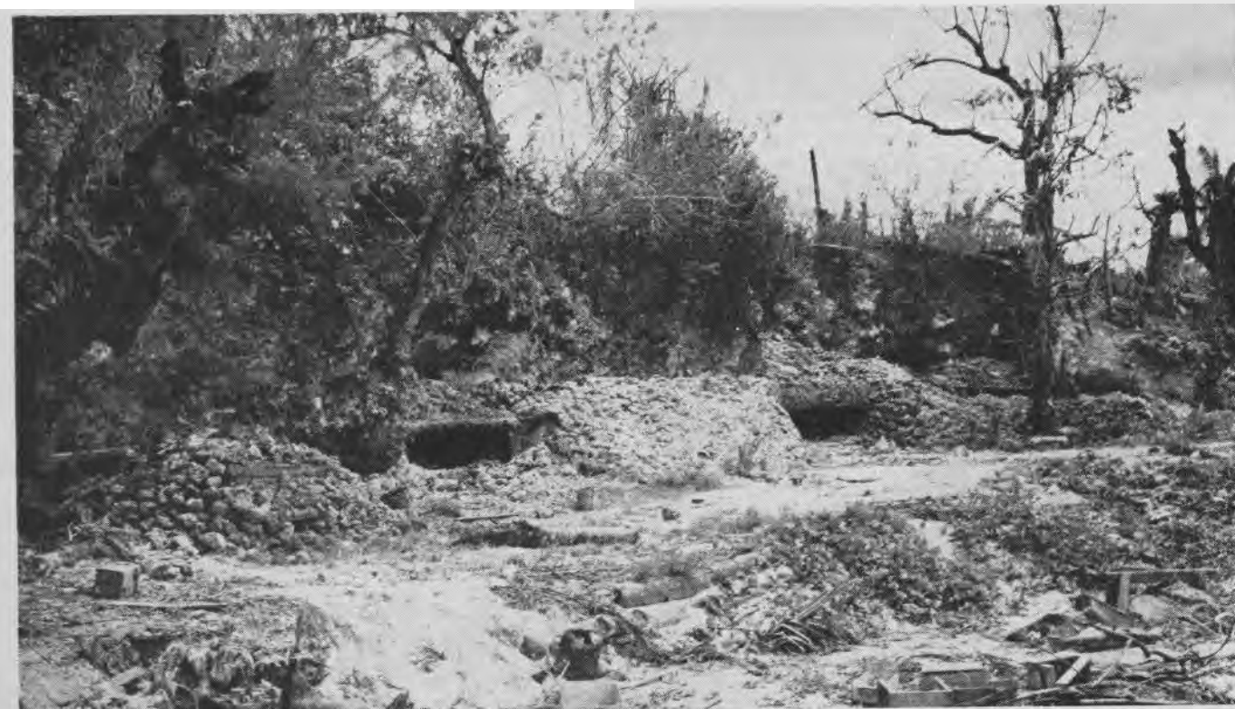
VIEW OF PILLBOX AND THREE GUN POSITIONS OF MASONRY BLENDED WITH CLIFF: LARGE CAVE DUG IN ROCK COVERS ARTILLERY AND SERVES AS QUARTERS
