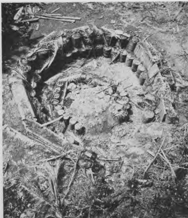
DOUBLE REVTMENTS AT AGAND GAIN STRENGTH FROM FUEL OIL DRUMS
