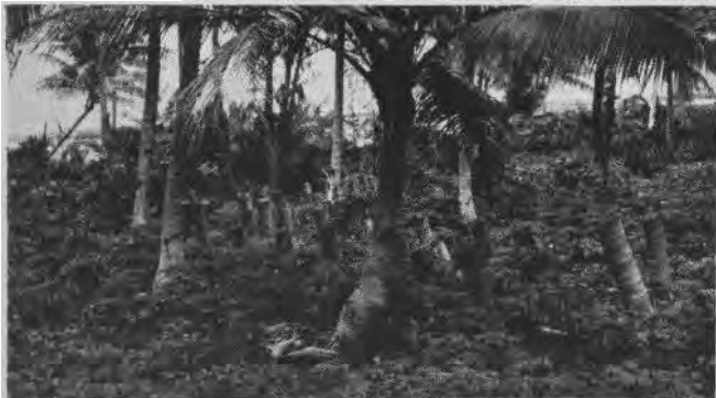
COCONUT LOGS FORM TANK BARRIER WITH LOW SHRUBS FOR CAMOUFLAGE
