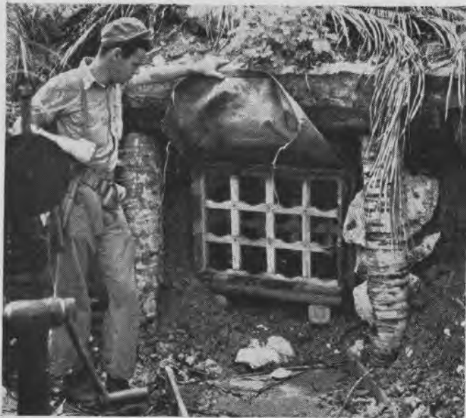
Marine holds up canvas cover of ammunition rack built into side of earth-covered revetment for 4.7" gun. Note log reinforcement
