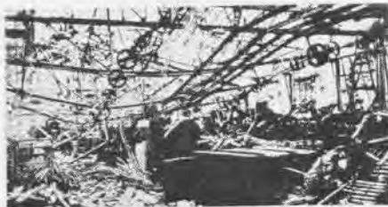
DEVASTATION OF MACHINE SHOP FOLLOWS RAID
