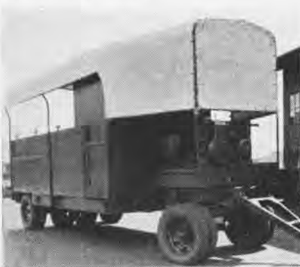
PEARL HARBOR BUILDS PRESERVATIVE TRAILER
