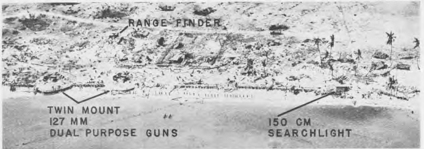
Closeup view of dual-purpose battery along the beach at Tarawa, showing relation of searchlight to battery; a similar light position on the other flank of the battery does not show in this photo; searchlight is on right and five-inch guns are on left
