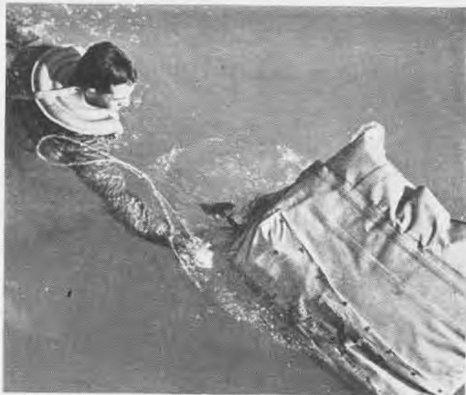
3 Life raft can be opened from the water by pulling the carbon dioxide release handle. Raft will drift fastest when inflated
