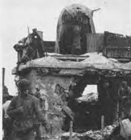
In spite of terrific pounding, this 150 cm. searchlight is still standing on the beach at Tarawa; sturdy base housing generator, hit by shell, exposes structure
