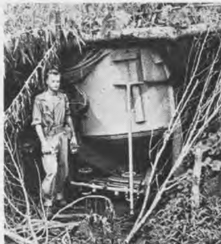
Camouflaged searchlight is concealed under shelter made of logs and natural growth; shelters built adjacent to revetments with an opening for concealing from view
