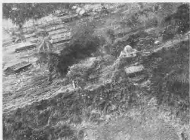
Oblique of a 150 cm. searchlight at Rabaul shows it mounted in a circular sandbag and wood revetment with generator underneath it
