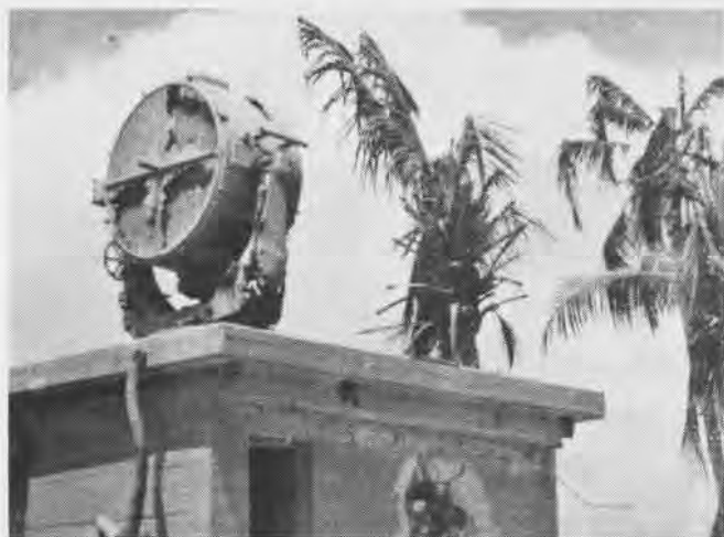
At Tarawa, this was one of two 150 cm. searchlights located 100 yards on each flank of two-gun twin mount five-inch gun battery
