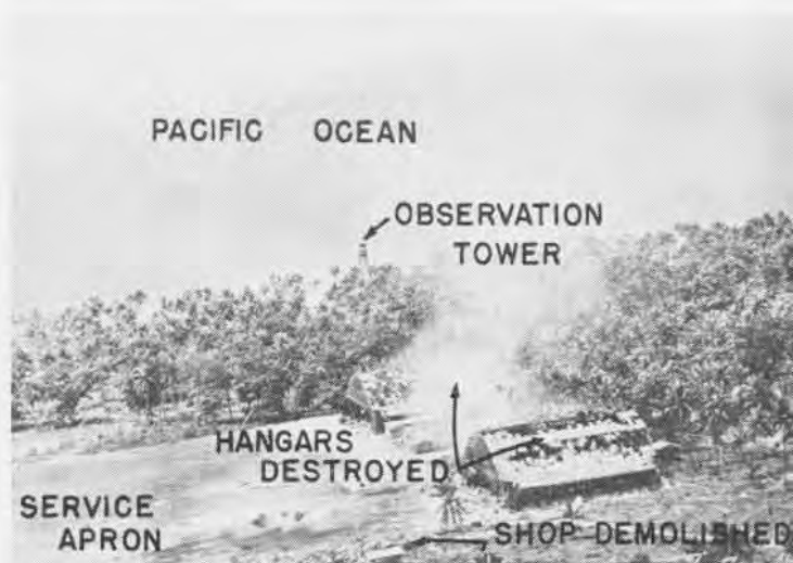
Low oblique covering detail in photo at farthest right shows demolition of hangars and repair shops. Bombs punched deep craters in service apron
