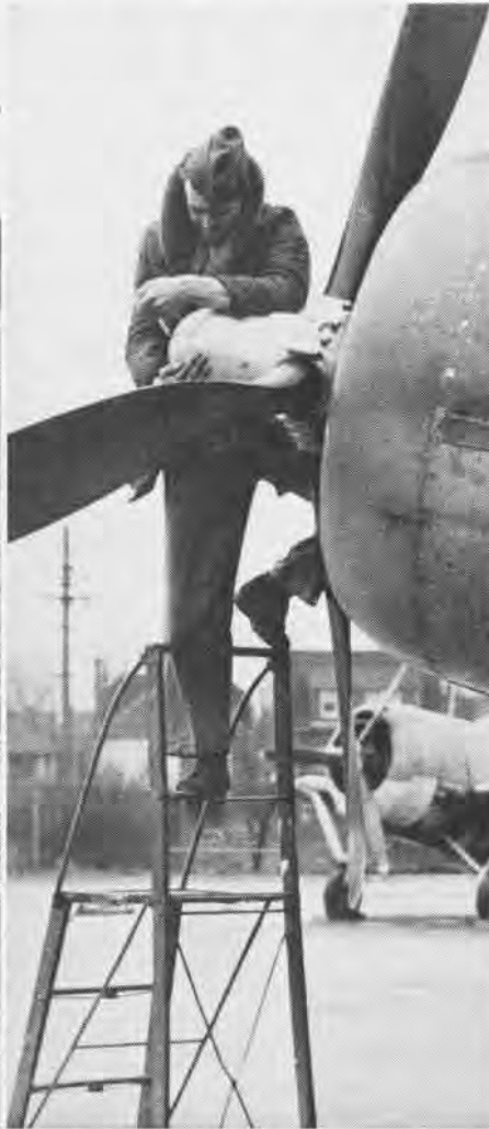
Propeller specialists learn maintenance and overhaul procedure as well as ground adjustment, testing and trouble shooting
