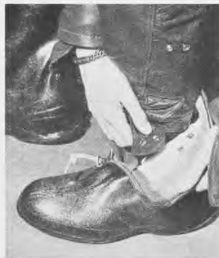
SNAPS CONDUCT CURRENT TO AVIATOR'S BOOTS
