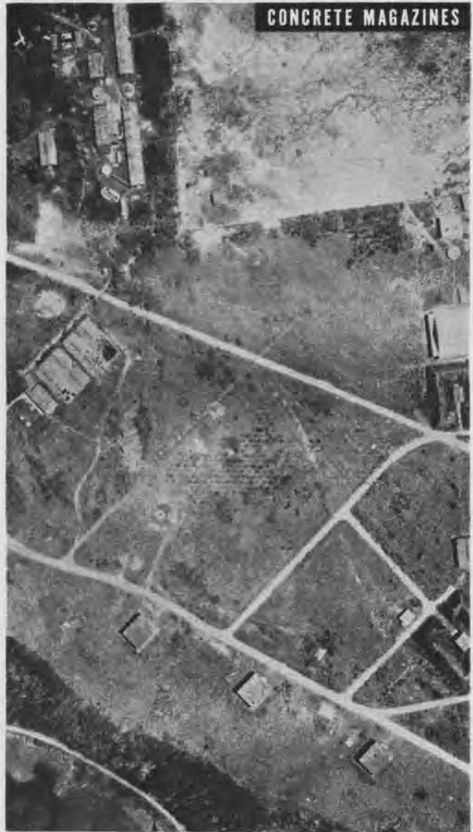
Typical layout of concrete storage buildings photographed at Saipan shows conspicuous shadows of structures along roadway
