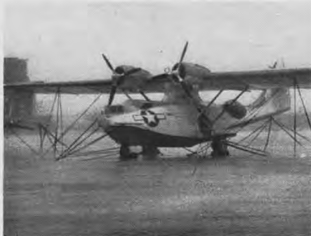
Secured In Accordance with established naval storm bill procedure, this Catalina went through hurricane at NAS Norfolk undamaged.
