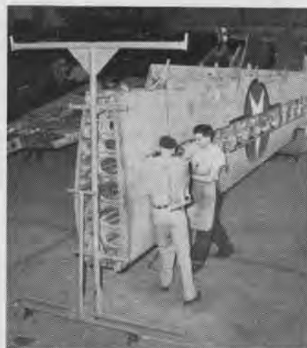
UNIVERSAL FIXTURE BOLTS TO THE WING ROOT
