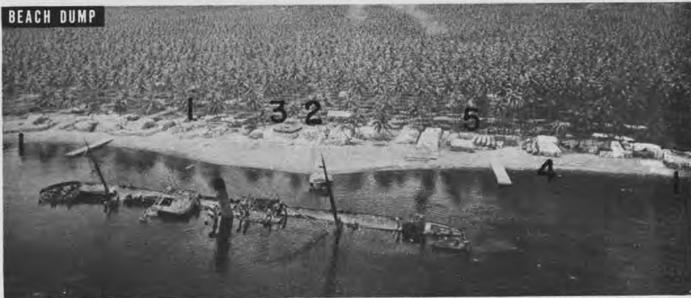
Sunken Keffuku Maru marks a typical beach supply dump for loose stores at Vunapope. This type dump is a distributing center
