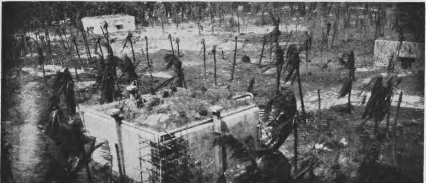
Two types of concrete storage buildings are shown here. Square structure in foreground with three ventilators and sod-covered
