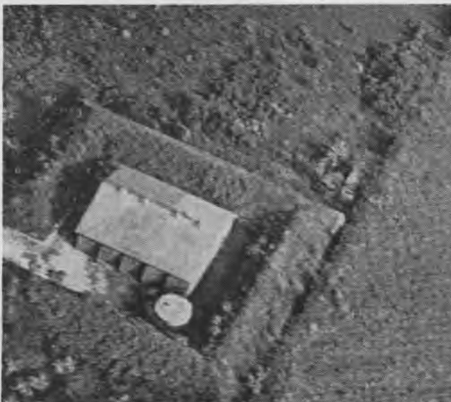
Explosive storage building, 50' x 50', probably for bombs at Aslito field, Saipan, is protected by heavy revetment of reinforced earth
