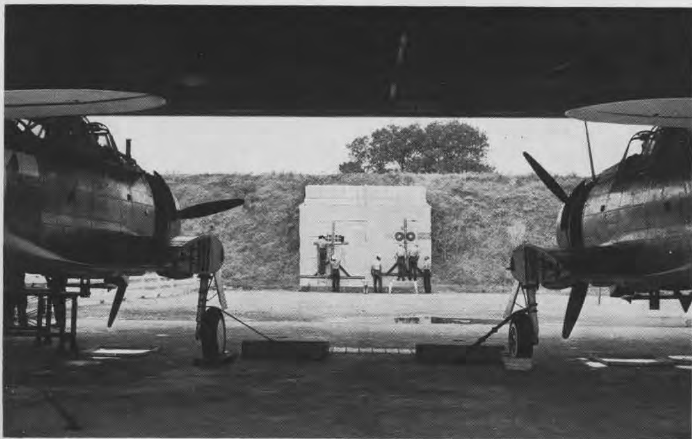
Boresighting guns is one of the jobs AOM trainees learn to do well during their training in operation group at NATC Norman. Students conduct rearming drills on F6F, F4U, SBD, TBF, SB2C, SB2U, PBV and other operational-type naval aircraft. Trainees get valuable experience installing ordnance gear, synchronizing guns, rearming aircraft with various type loads, and range firing.
