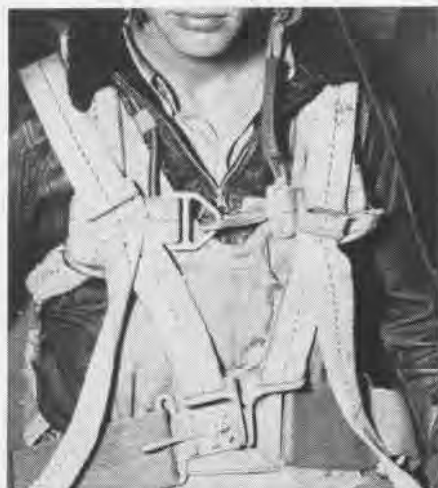
WEB STRIPS COMPRISE THE SHOULDER HARNESS
