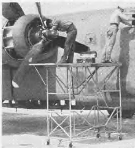
PLATFORM CAN BE EXTENDED TO SERVICE PB4Y
