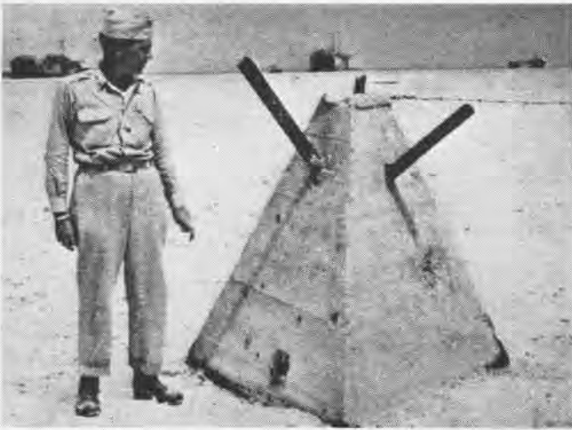
Pyramidal barricades have a triangular arrangement of steel beams set in concrete. These barriers form the outer defenses of islands
