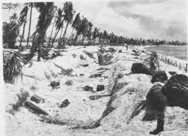
Tank ditch is located just inshore from the beach at Betio Island. Just beyond, barbed wire fences protect beach from invading troops
