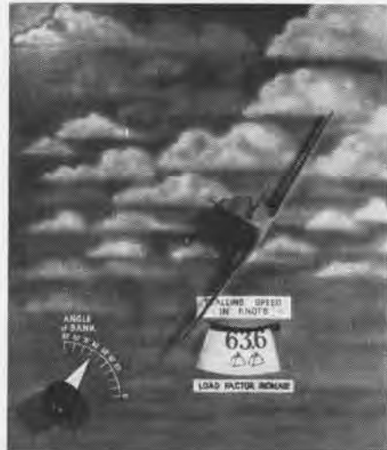
Memphis device demonstrates stall speed of aircraft with various banking angles
