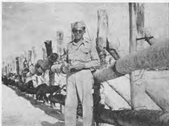
Close-up of seaward side of antiboat barrier made of logs in the shallow water of Betio beach. High tide raises water three feet
