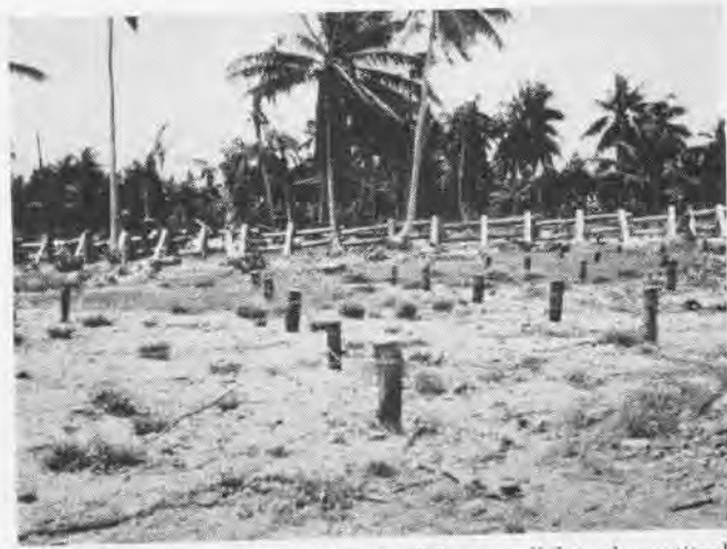
Low wire entanglement on Makin Atoll lies parallel to the antitank barrier in background. It usually forms a band 12 to 30 feet wide
