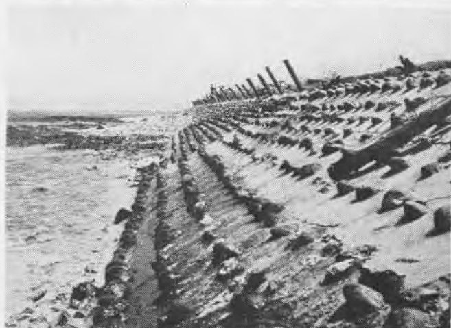
Permanent type of sea wall construction is built by the Japanese with boulders set in concrete and barbed wire fence along the top
