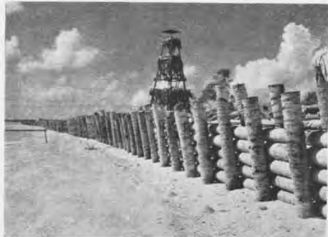
Japs took this photo of a completed coconut log barricade in the form of a sea wall along beach. Shows use of materials at hand
