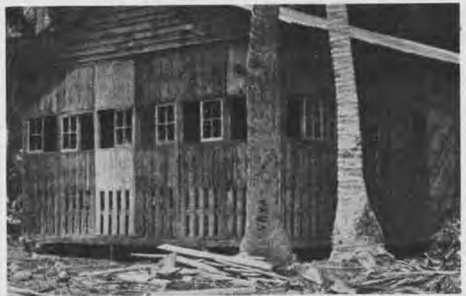
STORAGE BUILDING IS MADE OF PREFABRICATED WOODEN PANELS
