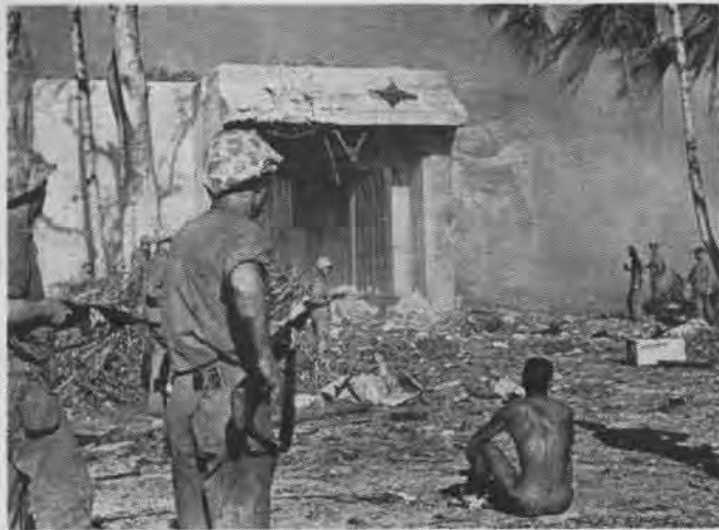
OVERHEAD LOADING TRACK SHOWS IN PORCH OF AMMO STRUCTURE
