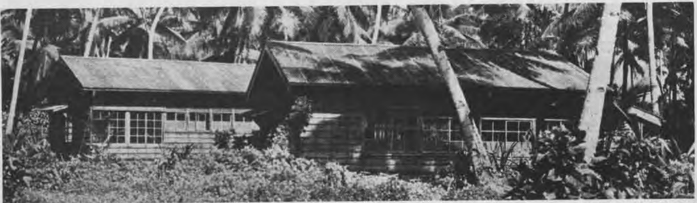
SHED IN REAR OF BATH HOUSE CONTAINS TWO HOT WATER HEATERS AND HAS STACK WHICH SOMETIMES IS VISIBLE FROM THE AIR
