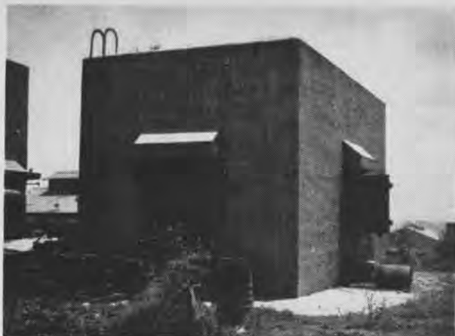
SPECIAL OIL STORAGE STRUCTURE IS IN POWER PLANT GROUP
