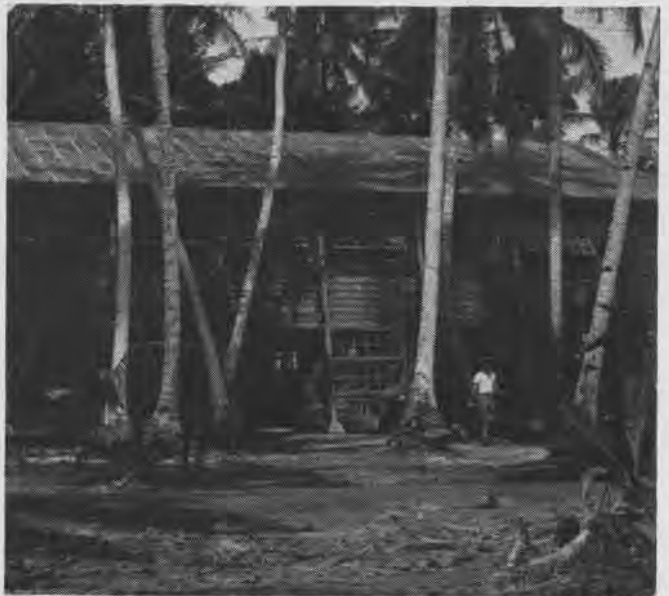
REPAIR HANGAR IS GABLE-ROOFED WOOD FRAMED STRUCTURE
