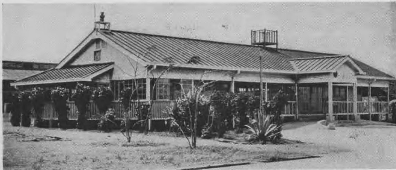
AIRFIELD ADMINISTRATIVE ACTIVITIES ON SAIPAN WERE CONDUCTED IN THIS ONE-STORY GABLE-ROOFED WOOD FRAME BUILDING
