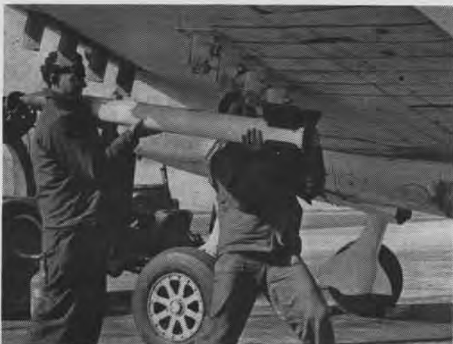
Assembled rocket is inserted on the launchers, the rear release pin is cocked and the round secured. Earlier model of launcher has shear pins, which had to be installed prior to final plug-in so the rocket would not drop off while diving
