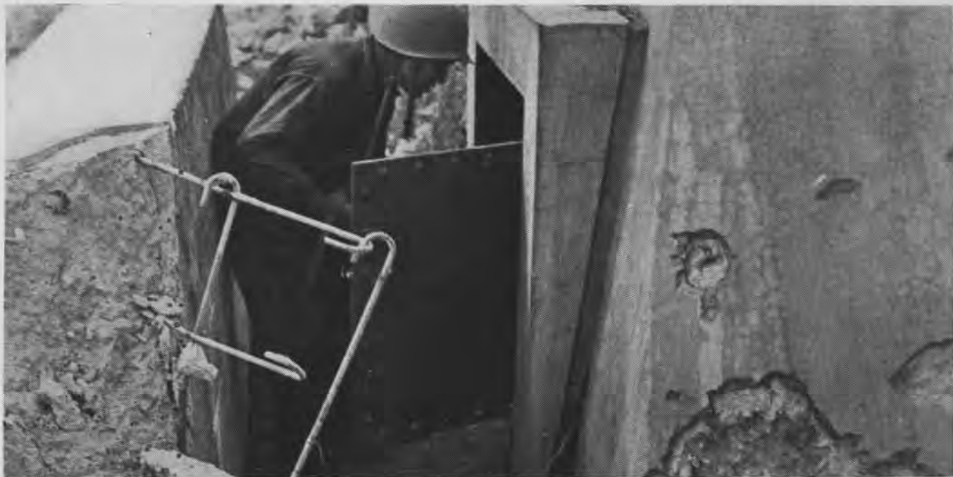
DOUBLE VAULT DOORS. WHEN PROPERLY OPERATED, MAKE JAPANESE AIR RAID SHELTER GAS-PROOF. NOTE ANTI-STRAFING WALL
