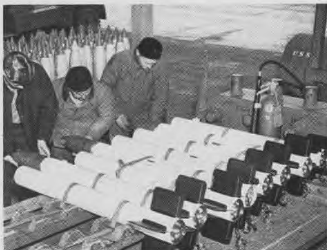
Rocket motors are carried by truck to another shed where the explosive heads are screwed on. Head must fit tightly to permit proper functioning of base fuze. Rockets are easily visible for photographic analysis studies when painted white
