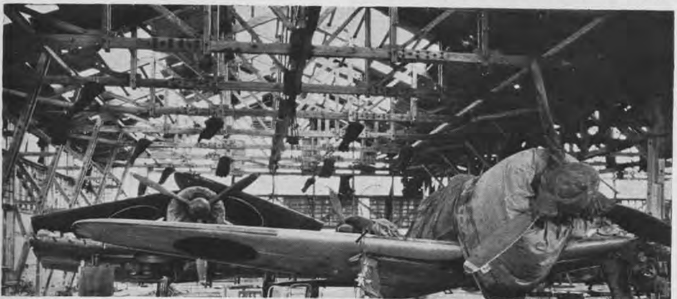
INTERIOR OF ENEMY'S HANGAR WORKSHOP ON SAIPAN IS WELL LIGHTED. BEAMS AND OTHER SUPPORTING MEMBERS ARE OF WOOD
