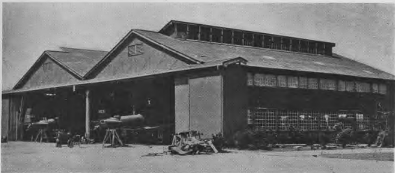
WOOD FRAMED HANGAR WORKSHOP HAS DOUBLE RIDGE ROOF. DOOR TRACK EXTENDS 15 FEET BEYOND THE BUILDING ON EACH SIDE
