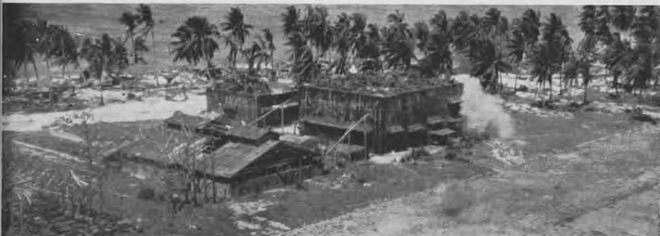
THIS POWER PLANT WAS ON WOTJE. SHOP AT EXTREME LEFT IS WRECKED, AND BOMB HAS PIERCED ROOF OF WATER-COOLING TANK
