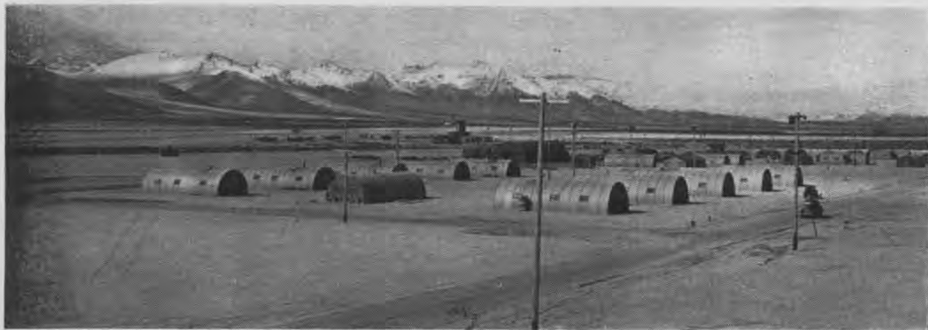
QUONSET HUTS, LANDING STRIPS AND SAND COMPRISE HARVEY FIELD, NEAR INYOKERN, WHERE PLANES FLY OUT TO TEST ROCKETS
