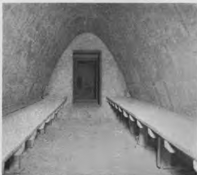
INTERIOR HEIGHT IS FIVE FT. SHELTER HAS THREE ENTRANCES
