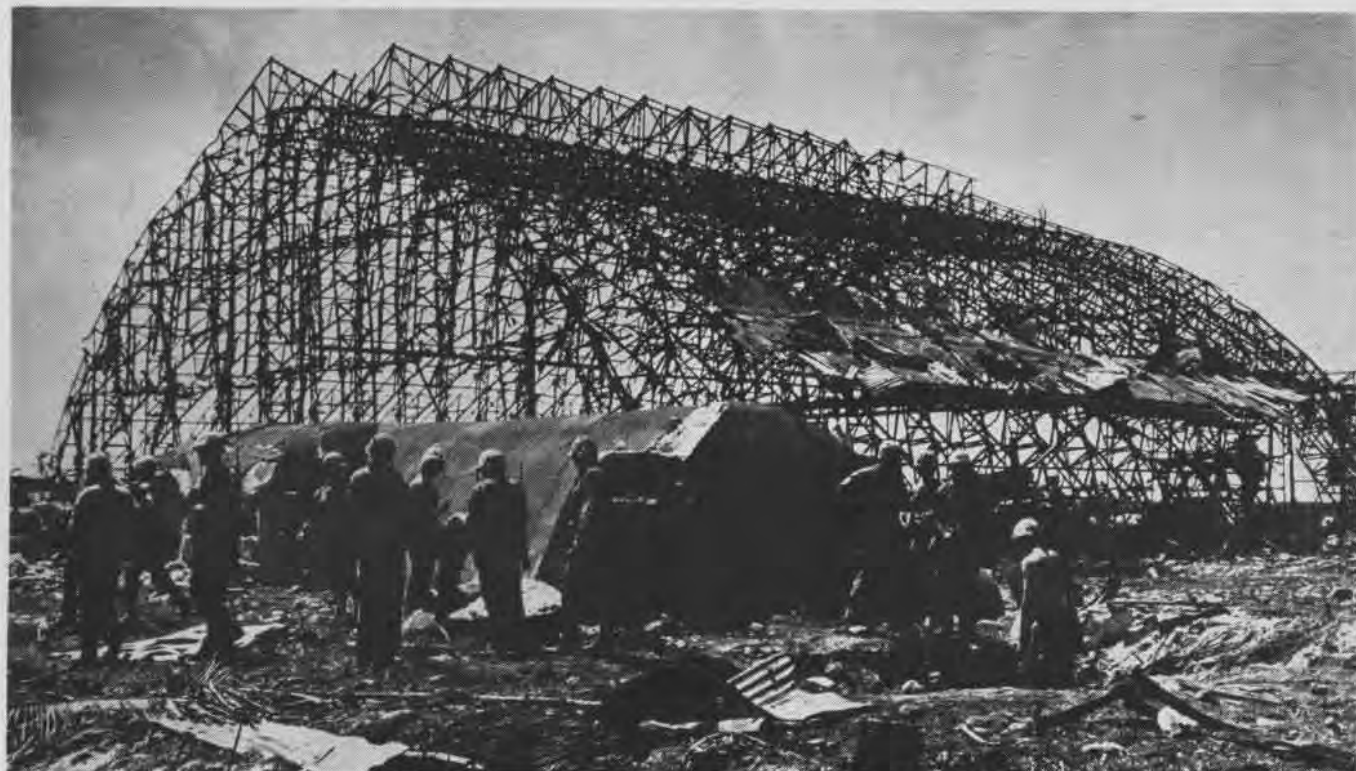
STEEL FRAMEWORK OF ARCH-ROOFED JAP HANGAR STILL STANDS ALTHOUGH CORRUGATED IRON SURFACING HAS BEEN BLASTED OFF
