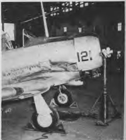
STAND HOLDS PLANE NOSE DURING REPAIRS
