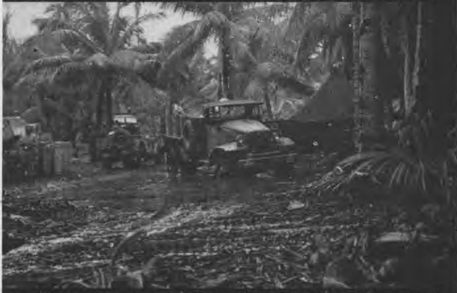
TROPICAL RAINS COMPLICATE SUPPLY, CONSTRUCTION AND ADD GENERAL DISCOMFORT
