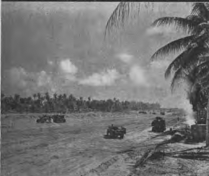
TRUCKS DUMP CORAL ON STRIP; SCRAPERS, BULLDOZERS SPREAD IT
