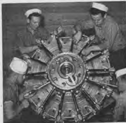
SHOP MECHS ASSEMBLE AN OVERHAULED ENGINE
