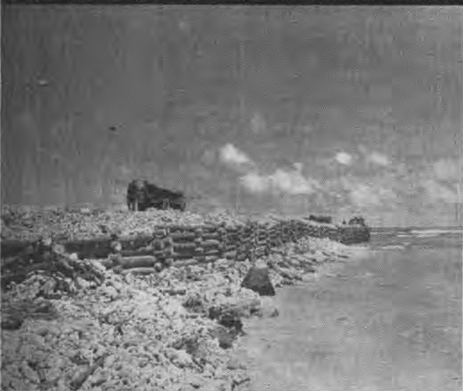
CORAL-FILLED CRIBBING PROTECTS WARM-UP APRON FROM THE SEA
