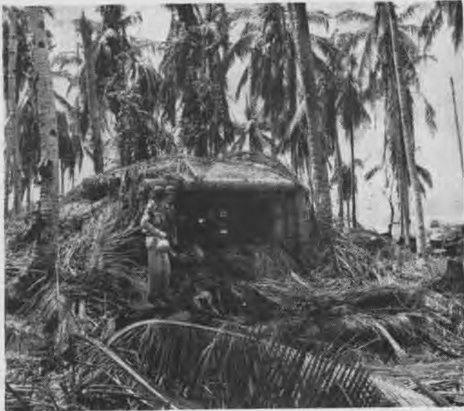
Typical 75 mm. gun position is well camouflaged with palm fronds reinforced with coconut logs. Gun can be quickly withdrawn
