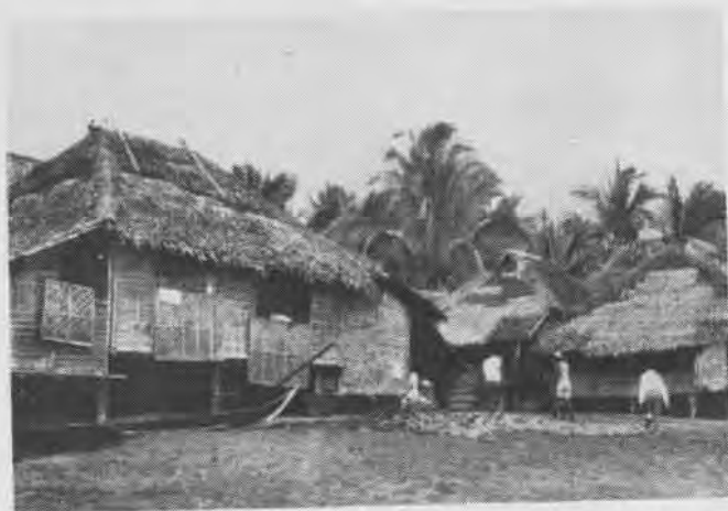
Native huts on Leyte show method of building with local materials and elevating houses on pilings. Roofs are thatched of palm
