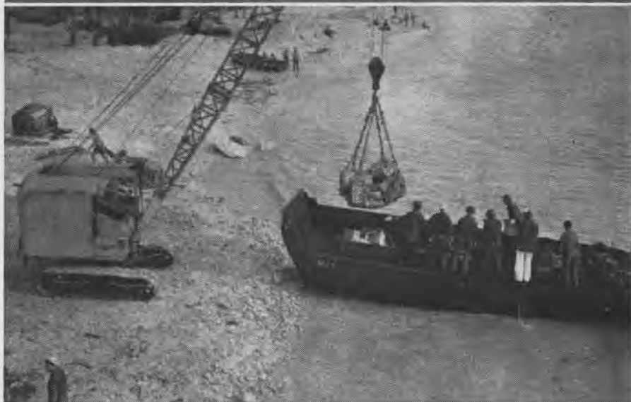
POWER CRANE UNLOADS LSV'S AND OTHER CRAFT, SWINGING AROUND TO LOAD TRUCKS
