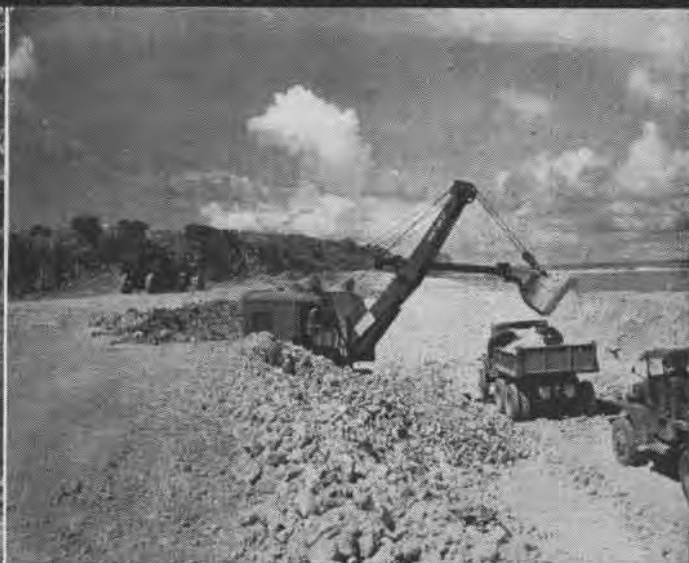
AT CORAL PIT ALONG SHORE, POWER SHOVEL LOADS STREAM OF TRUCKS
