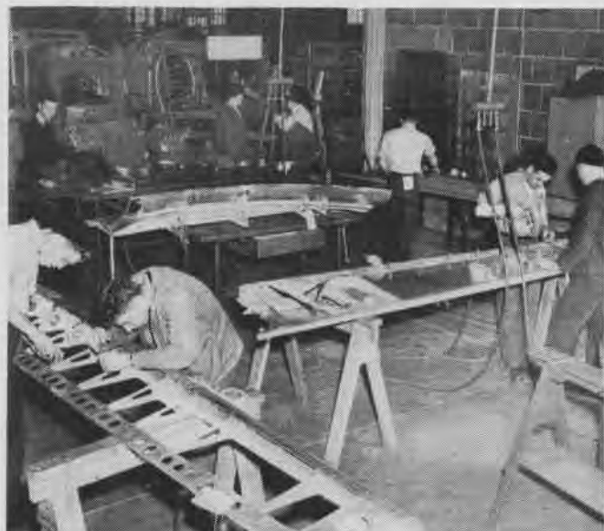
METALSMITHS AT ABATU, ST. LOUIS, REPAIR FLAPS AND AILERONS
