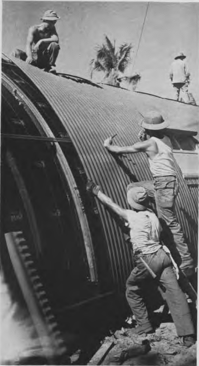
Seabees attached to ACORN on Eniwetok set up Quonset huts to house men at the base. Advanced areas lack palatial quarters
