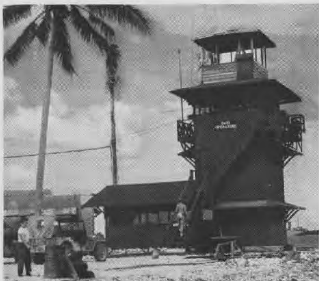
ACORNS BUILD AND OPERATE SUCH TOWERS AT SEAPLANE BASE
