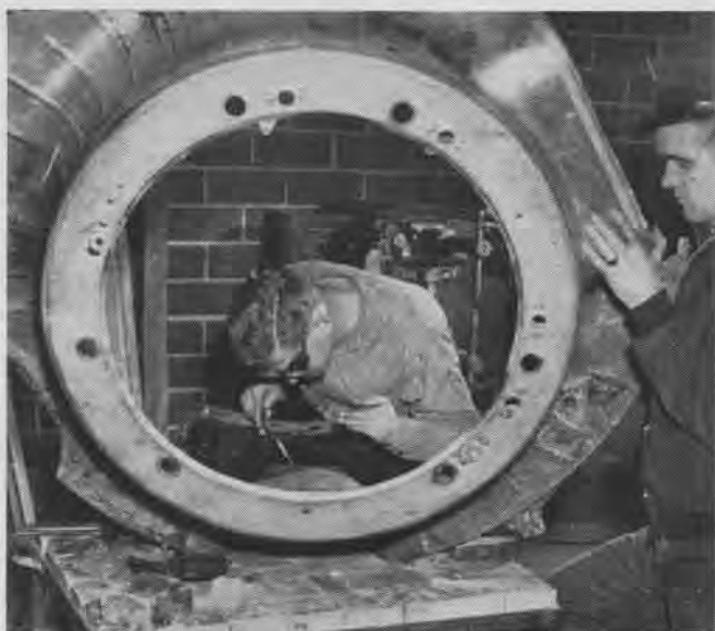
ABATU MECHANIC WELDS COWLING FOR PRACTICAL EXPERIENCE
