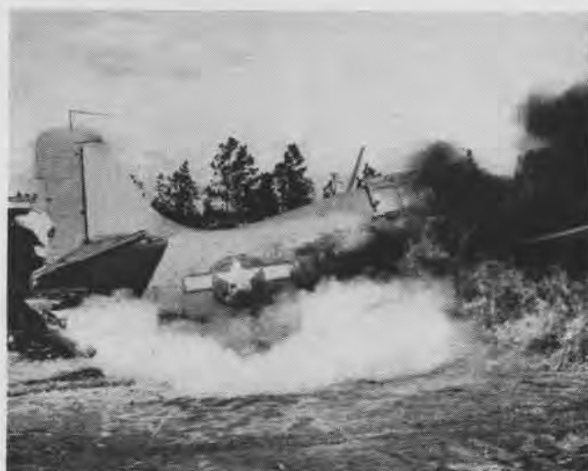
Carbon dioxide, released close to ground from discharge horns quickly smothers flame around gasoline spilling from wing tank
