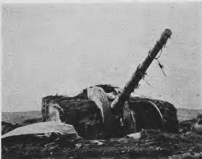
Sometimes, as at Kiska, Japanese install 120 ashore complete with shield, canopy. It usually has no shield when land-mounted
