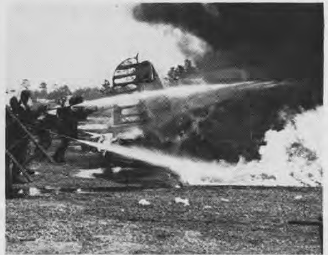
Crash fire rescue crews use two fog lines to protect cockpit and two for sweeping the runway clear of all the burning gasoline
