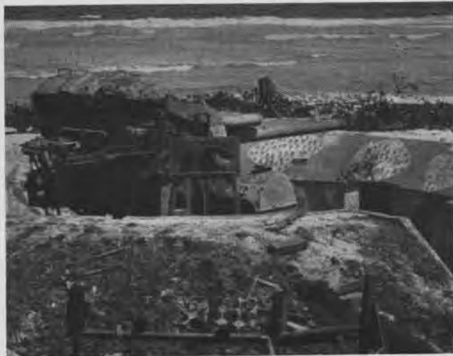
Twin barreled 127 is set on electrically operated pedestal mount. Concrete revetments have ready ammunition lockers set in walls
