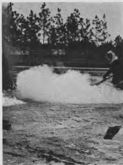
CO 2 BLANKETS FIRE FROM WING TANK SPILL
