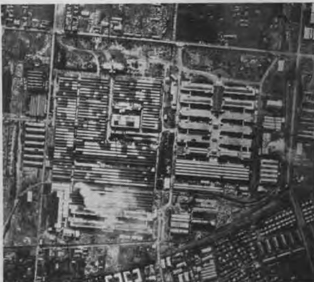
Nakajima Musashi Factory has fireproof, multi-storied buildings at right, with older, typical one-story engine shops on left
