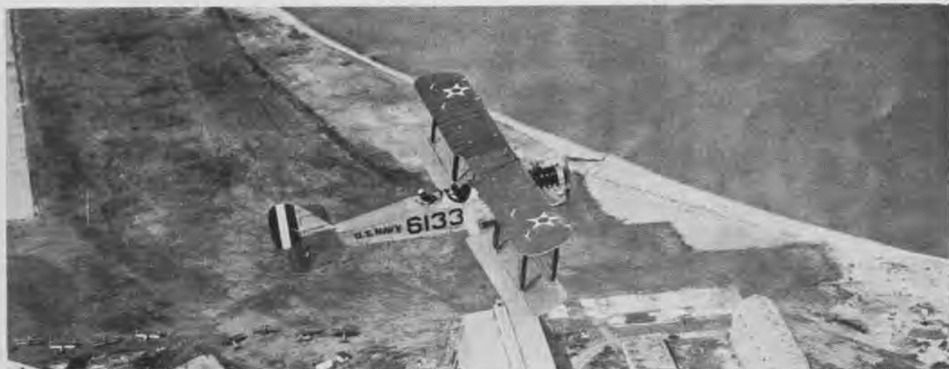
A DH-4 IN FLIGHT OVER NAS PENSACOLA. CONVERTED PLANES DID AWAY WITH SECOND COCKPIT LEAVING ROOM FOR BASKET LITTERS
