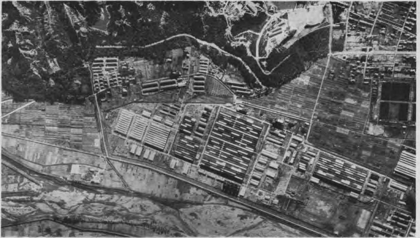
PART OF LARGE MITSUBISHI ENGINE WORKS AT NAGOYA. TEETHLIKE SHADOWS IN LOWER CENTER ARE CAST BY ENGINE TEST CELLS
