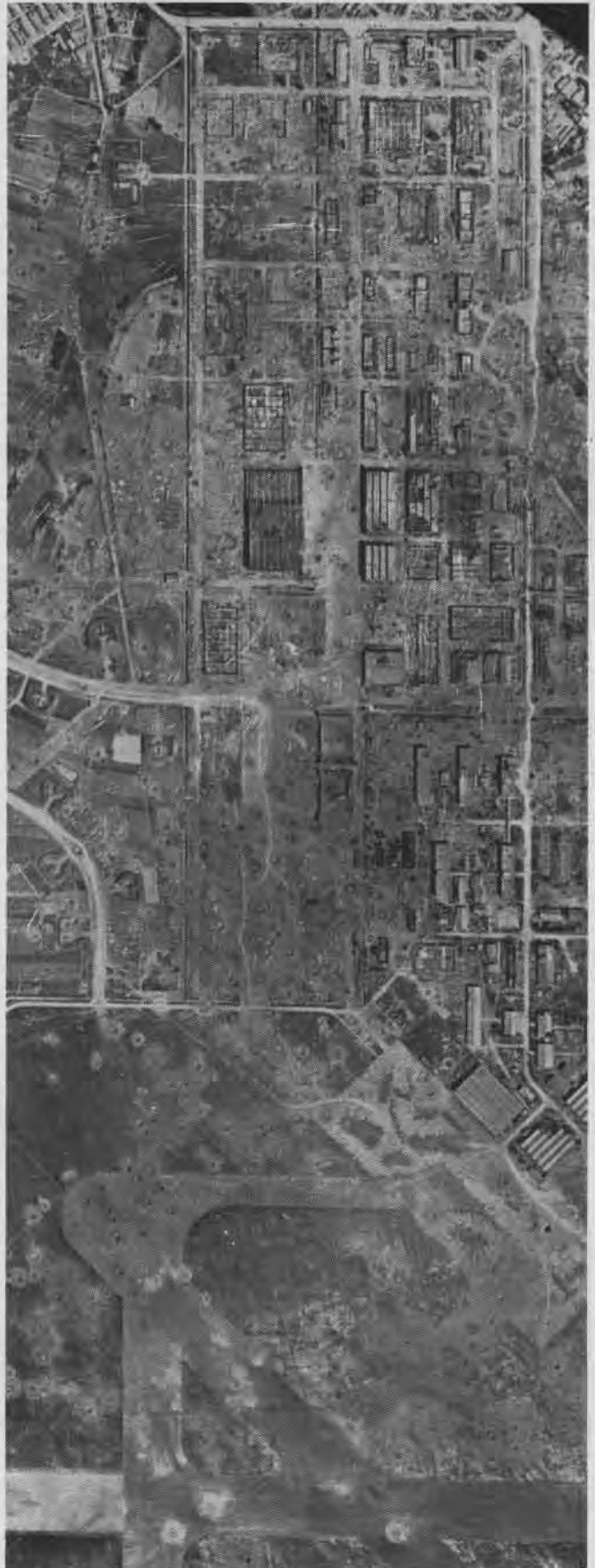
After Activity is halted completely by bombs from Army B-29's and carrier-based Navy planes. Many buildings of wooden construction burned to the ground. It is estimated that Japs will need four or five months to restore plant
