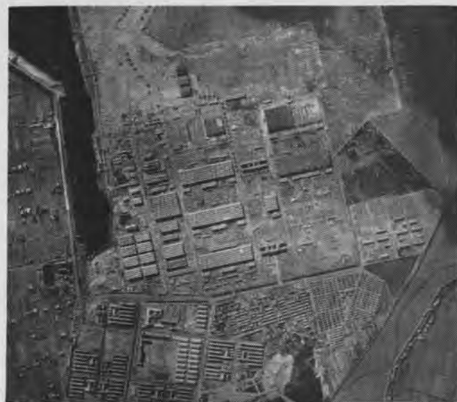
Finished Betty's are lined up at Mitsubishi Mishima plant. Tall completed building on right evidently is used for final assembly
