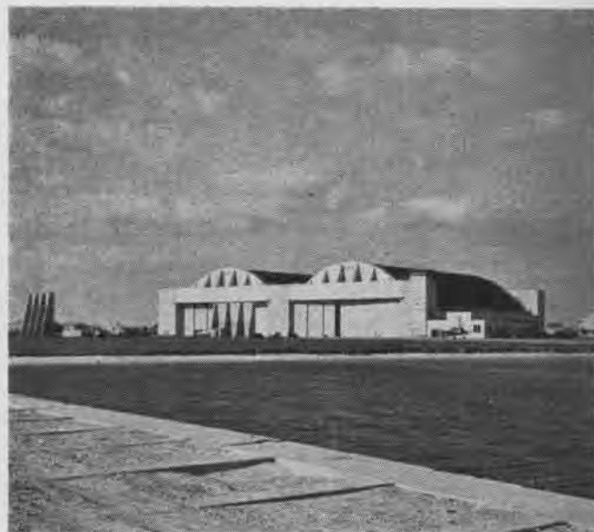
Armament Test hangar apron has facilities for ground-firing at either water or land targets like the large cement butt on the left
