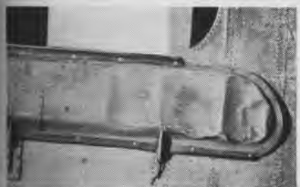
SPOILERS ARE CUT OFF BELOW BOTTOM HINGES
