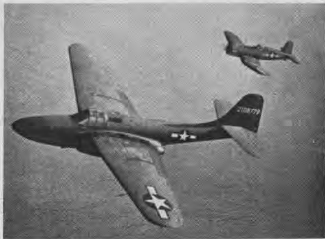
Late model Corsair , undergoing flight test, joins up with the propellerless YP-59-A jet propelled plane during experimental trial
