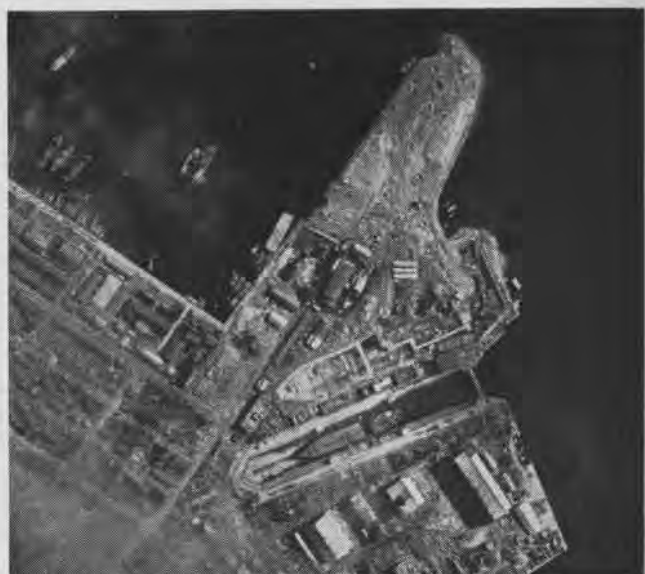
NEW DRYDOCK IS BEING BUILT AT KIURUN HARBOR, FORMOSA
