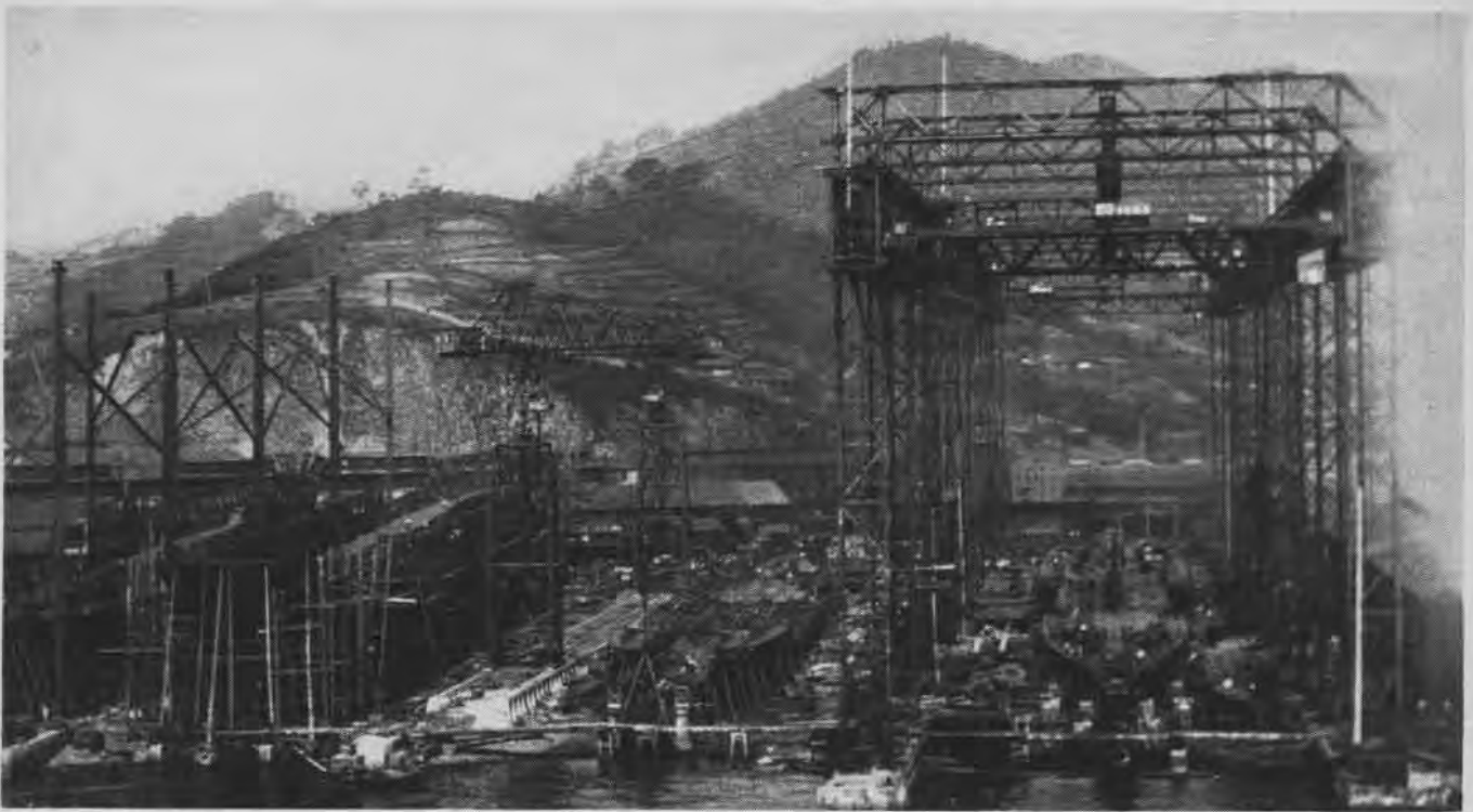
OLD PICTURE SHOWS BUILDING WAYS AND CRANES IN SHIPYARD AT NAGASAKI. HILLS IN BACKGROUND MAKE EXPANSION DIFFICULT
