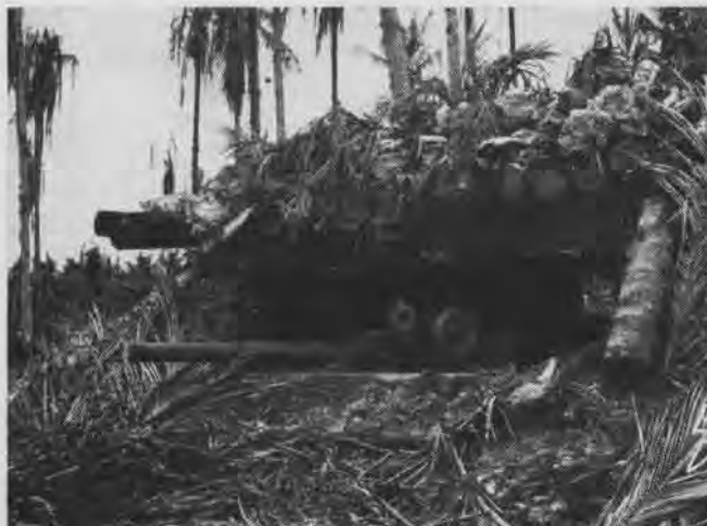
COCONUT LOGS AND ROCKS COVER THIS 76.2 MM. EMPLACEMENT
