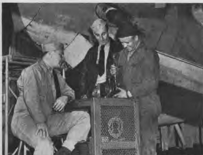
HANGAR DECK OFFICER CHECKS MECH'S WORK ON A MAGNETO
