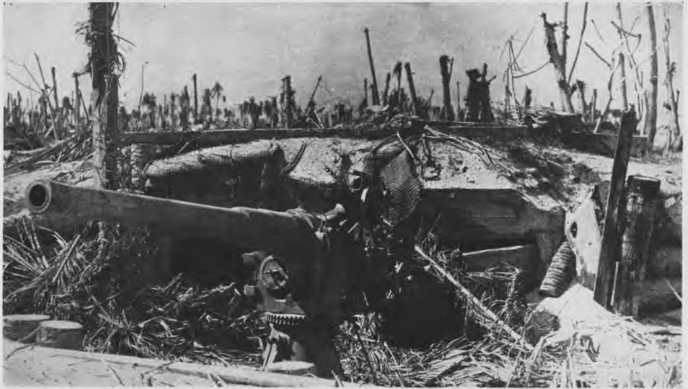
JAP 76.2 MM. COAST DEFENSE GUN WAS PURCHASED ORIGINALLY FROM BRITISH FACTORIES. THE GUN IS POINTED AND RAISED BY HAND
