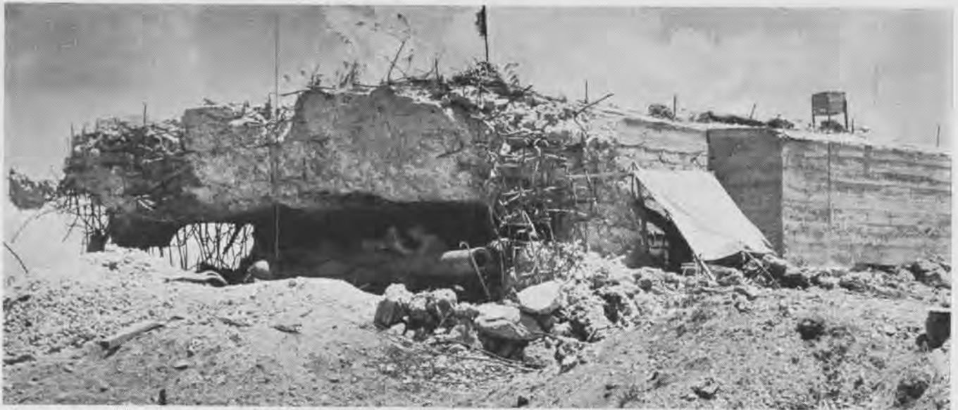
HEAVY REINFORCED CONCRETE EMPLACEMENT COVERS JAP 150 MM. COAST DEFENSE GUN ON SAIPAN, MAKING IT A DIFFICULT TARGET
