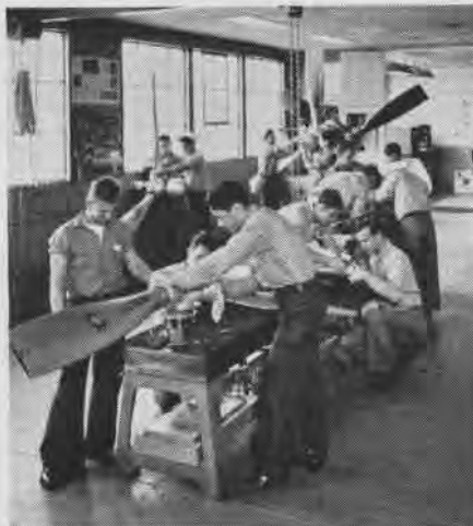
Students disassemble and adjust Hamilton hydromatic propeller, and work on electrics
