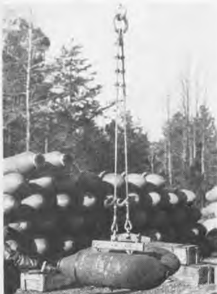
USE CABLES FULL LENGTH WITH CARRIERS
