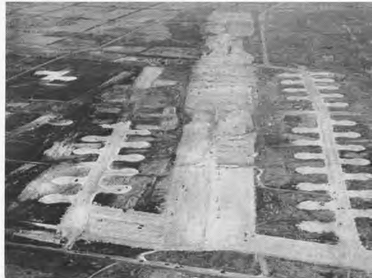
Construction work was still going on at this giant Tinian airfield when photo was taken; island later had 39 miles of runway
