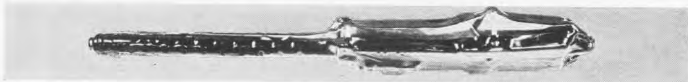
4 Dipping completed, the guns are hung up to dry. Protection will last as long as a year. Coating exudes oil which protects enclosed gun
