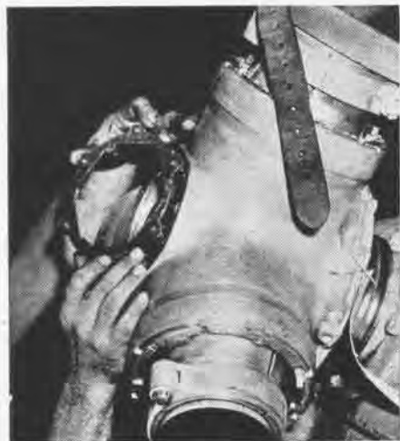
GEAR TEETH ALIGN WITH FLANGE POINTS
