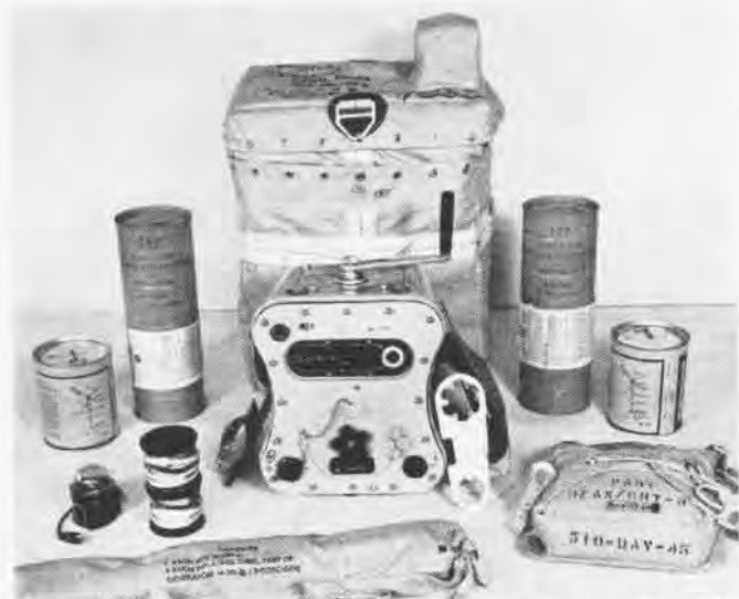
NEW GIBSON GIRL, AN/CRT-3, HAS MORE RANGE, CLEARER SIGNAL
