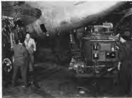
QUONSET'S TANK RESEALING PLAN WORKS
