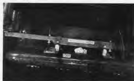
BOMB RELEASE GEAR HOOKS ON SCAR RACK
