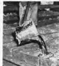
POURING BY HAND
