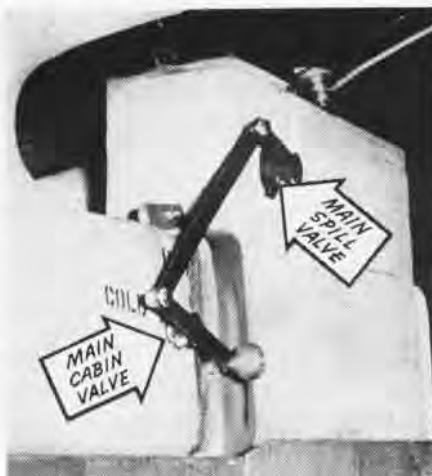
CORRECT INSTALLATION OF HEATER GEAR
