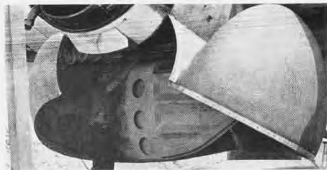
OPEN JAWS OF AN/APS-20 RADOME REVEAL BIG ANTENNA SCANNER
