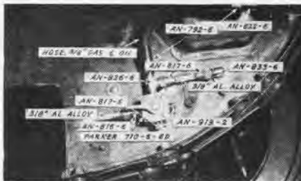
INSTALLATION DRAWS MOISTURE FROM OIL
