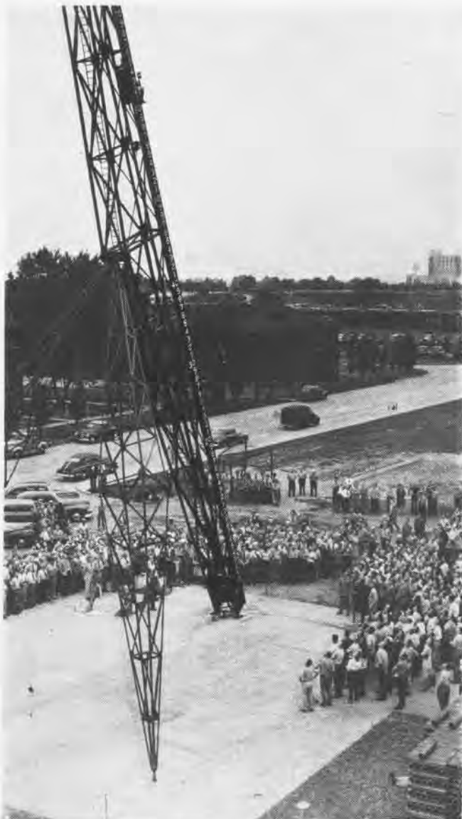
TEST TOWER AT NAMC, PHILADELPHIA. BLOWS MAN 73 FEET UP
