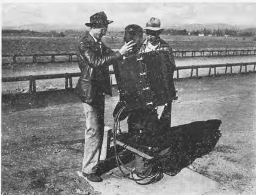
POWERFUL APPROACH LIGHTS PERMIT BLIND LANDINGS AT EXPERIMENT STATION, ARCATA
