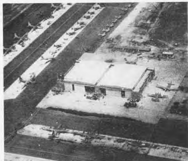
Spacious parking ramps and well equipped shops simplify operation of various types of training aircraft based at Whiting Field
