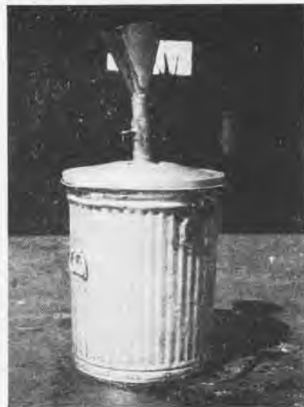
DRAINAGE CAN FIXTURE STOPS OIL SPRAY
