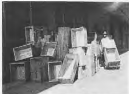
SPARE BOXES PILED READY FOR REUSING
