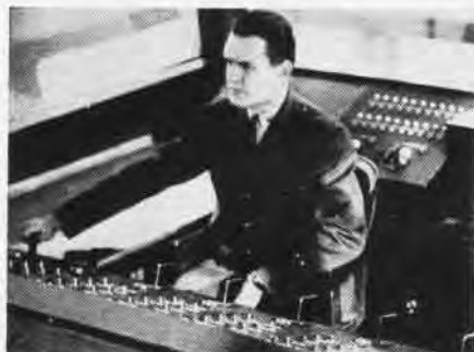
CENTRAL CONTROL OPERATES ALL BURNERS
