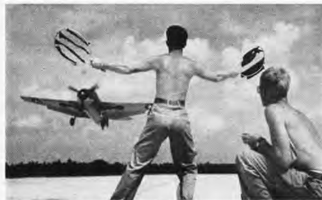
Pilots and flight deck crews train for carrier work on "field" carrier decks, complete with landing wires, barriers and an LSO
