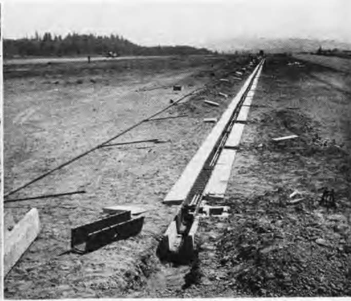
Slot Burner (Mk 5) gives 10 minute burn on 2500 gallons gas; British now use this type burner commercially at Heathrow field
