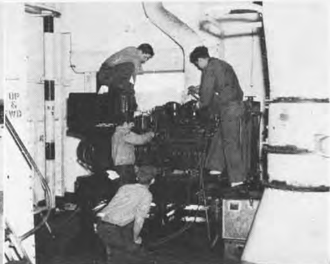
Workers secure an auxiliary engine on the hangar deck, spraying a preservative coating over it; machinery is always ready to run
