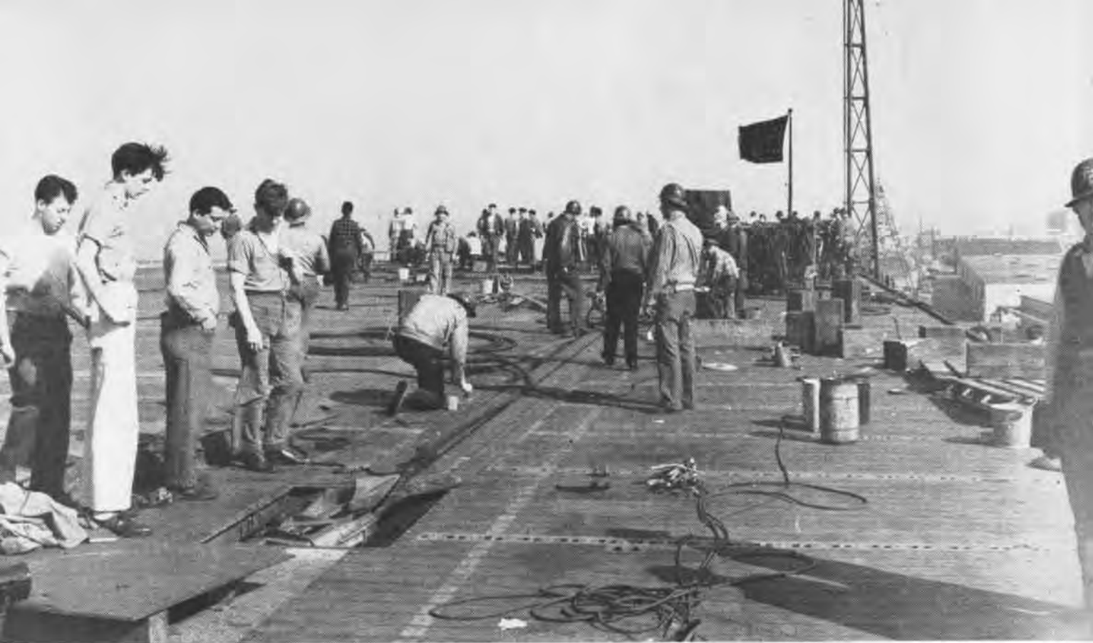
ONE OF THE MANY DECK JOBS ABOARD THE WASP AFTER SHE REACHED BAYONNE WAS TO OVERHAUL AND RECONDITION HER CATAPULTS
