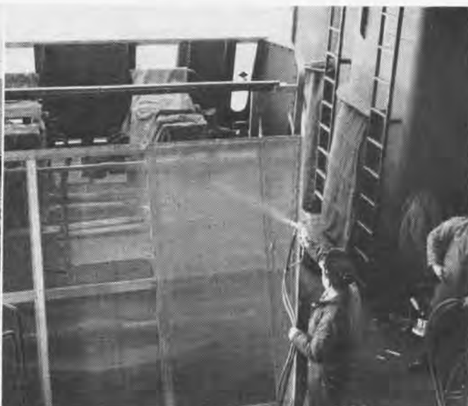
Quadruple mounts of 40 mm's are encased in framework and plastic webbing sprayed over it all; dessicants keep the inside dry
