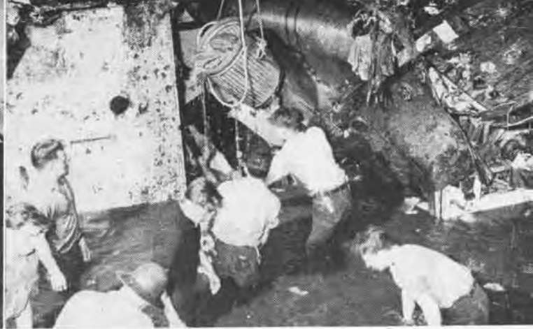
REPAIRING DAMAGE TO FOURTH DECK AFTER WASP'S ONLY 'HIT'
