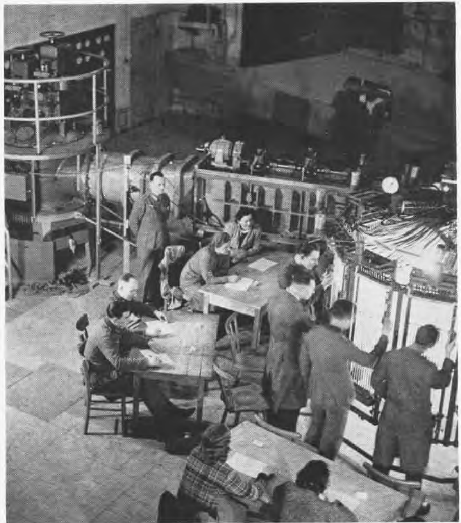
German photo shows technicians taking pressure readings from supersonic wind tunnel used in all experiments leading to V-2 rocket; captured tunnel is at NOL Washington
