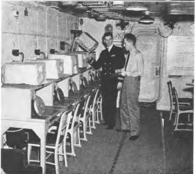
Two photos above are 'before' and 'after' shots of Wasp's radio room; sets wrapped in paper and room is given dehumidification
