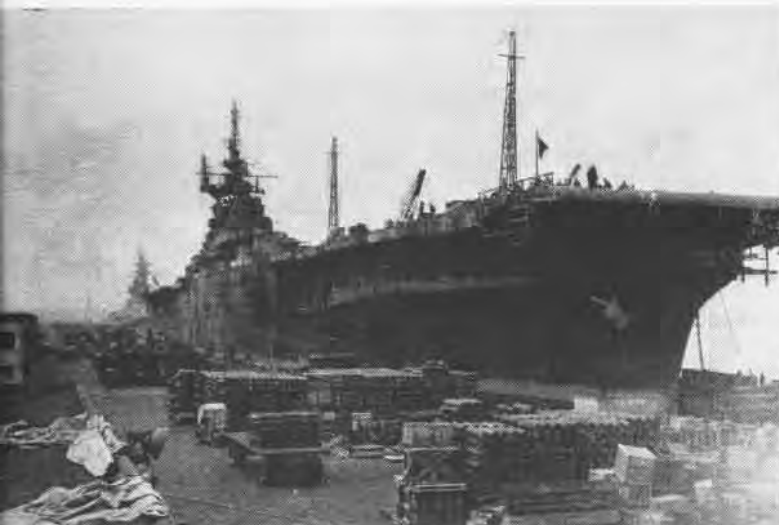
Wasp lies alongside its permanent berthing pier at Bayonne, awaiting preservation; oxygen containers used to repair storm damages
