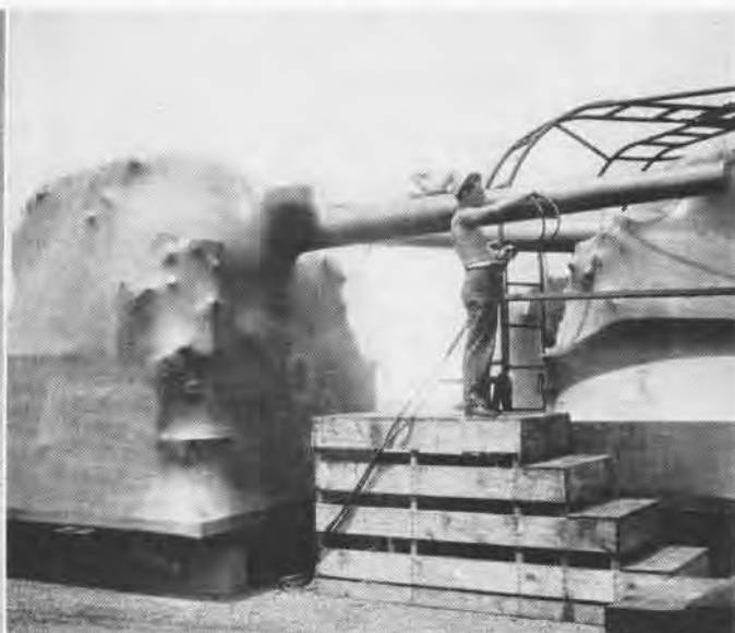
Spray man applies finishing touches of strippable coating to a dismantled 5" gun and mount, one of eight a typical CV carries
