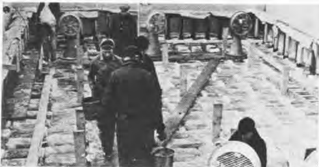
THIS GIANT "iceberg" carrier was considered by the Allies in the early part of the war as an antidote for the German submarine warfare and as a possible frozen airfield to provide cover for the invasion of
