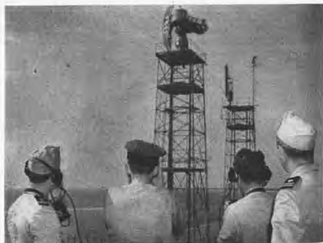
Atop the tower at King and Prince student officers guide planes in on visual intercept. Note CXHR radar antenna on tower
