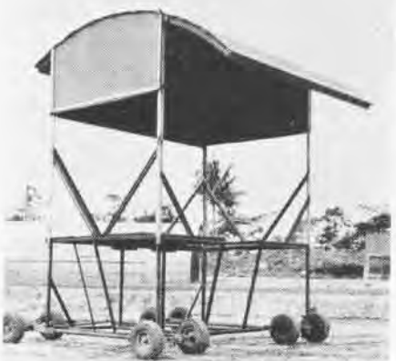
PORTABLE NOSE HANGAR HAS DROP CURTAIN
