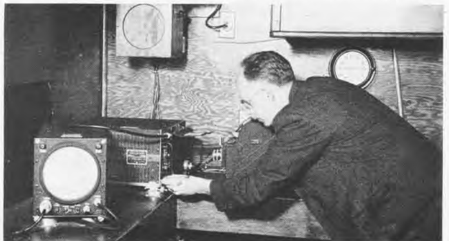
Permanent record of test flights is kept by movie camera focused on a television screen which provides more reliable data than can be recorded by pilot-observers
