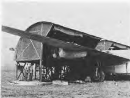
STATIONARY HANGAR HOUSES TWO ENGINES
