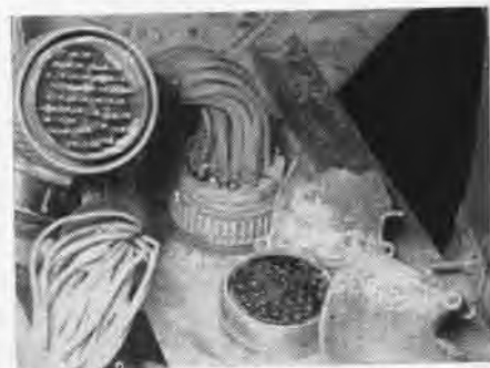
EXCESS MOISTURE CORRODES CONNECTOR
