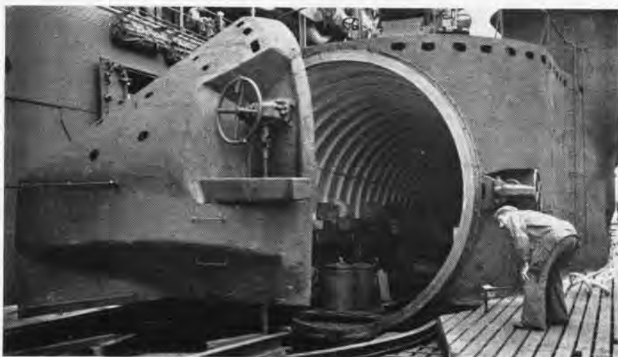
THIS IS TUBE OR HANGAR WHICH HOUSED THREE GLEN-TYPE FLOAT PLANES ON THE SUBS
