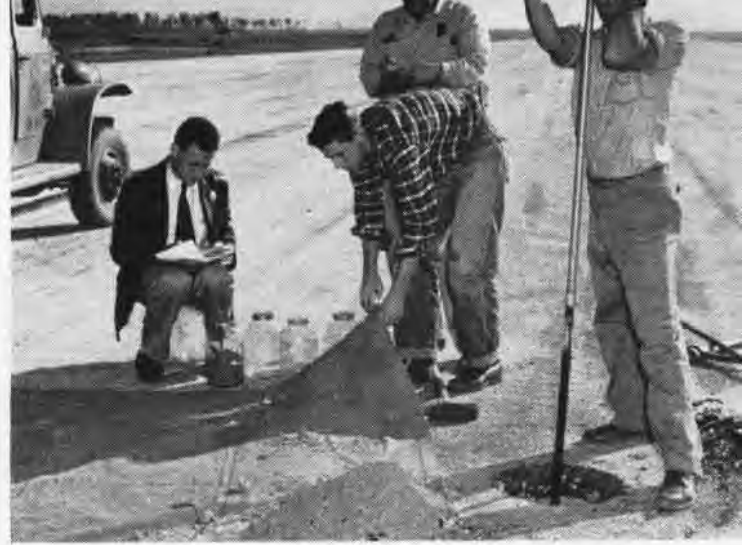
Soil survey crew make borings for samples every thousand feet on both sides of runways. Profile of airfield is plotted from data
