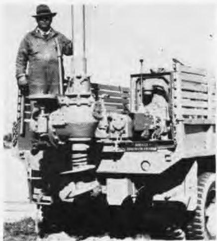
Evaluation program includes well digging; ground water elevation found with auger
