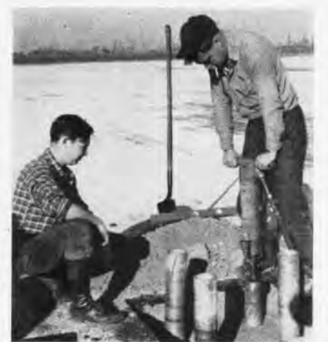
Material collected in tubes shows exact condition of subgrade after loading test
