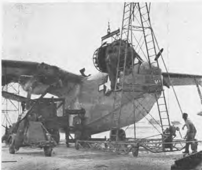
MECHS FIND JURY RIG HOIST USEFUL IN PBM-5E ENGINE CHANGE
