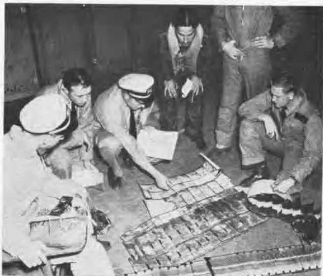
Instructor points out errors in mosaic taken by student division; Stereoscope viewer is visible on left, single recco strip at right
