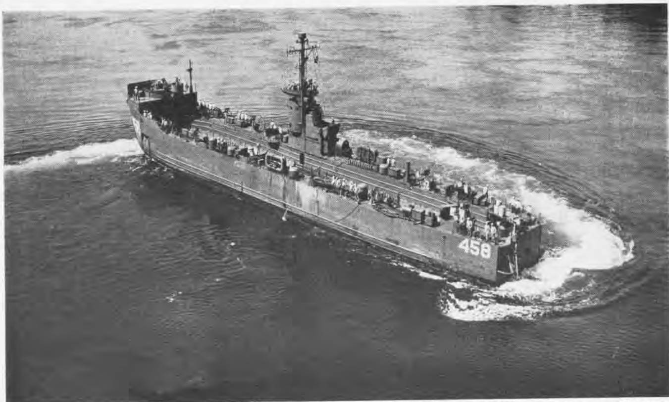
LSM-458, EQUIPPED WITH TWO CYCLOIDAL PROPELLERS, REVERSES DIRECTION QUICKLY IN MANEUVERABILITY TEST AT PUGET SOUND
