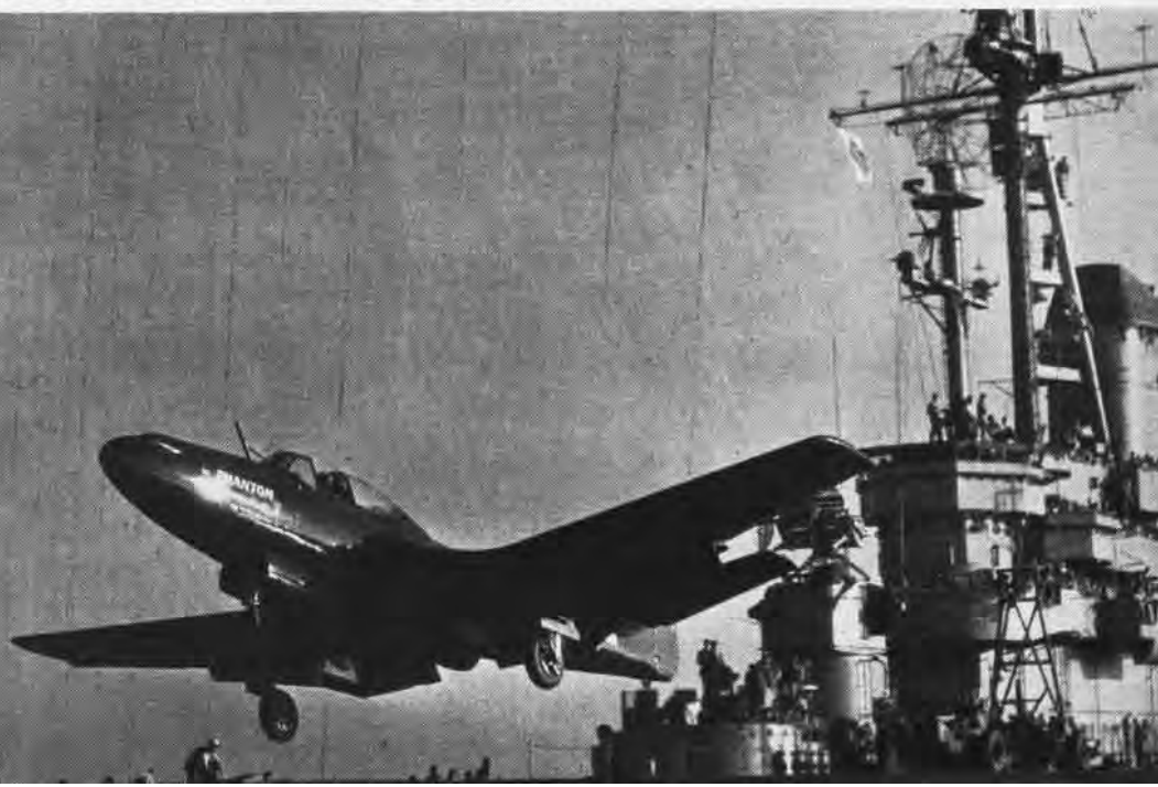
PHANTOM USED NO EXTERIOR POWER FOR TAKE-OFF DURING FIRST CARRIER TRIALS; HOWEVER, MOST JET PLANES WILL USE CATAPULT
