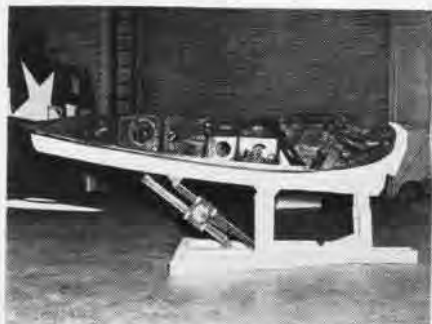
WING IN CRADLE ACCESSIBLE FOR WORK
