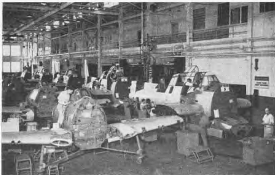
SPECIFIC JOBS ARE DONE ON SCHEDULE AT EACH SUCCESSIVE STAGE OF FUSELAGE REPAIR LINE
