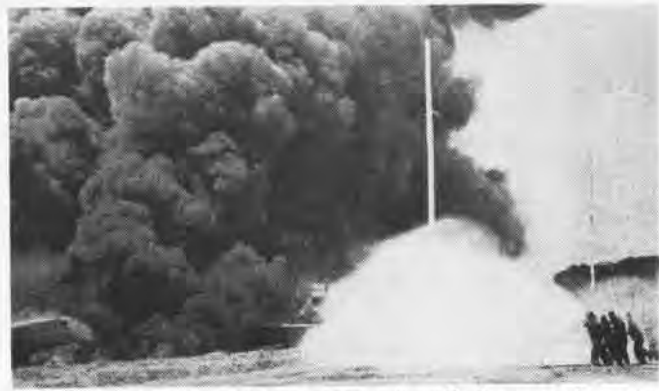
High capacity fire-fighting system installed on carriers gets a ground test; tugs also were given gear to combat oil fire
