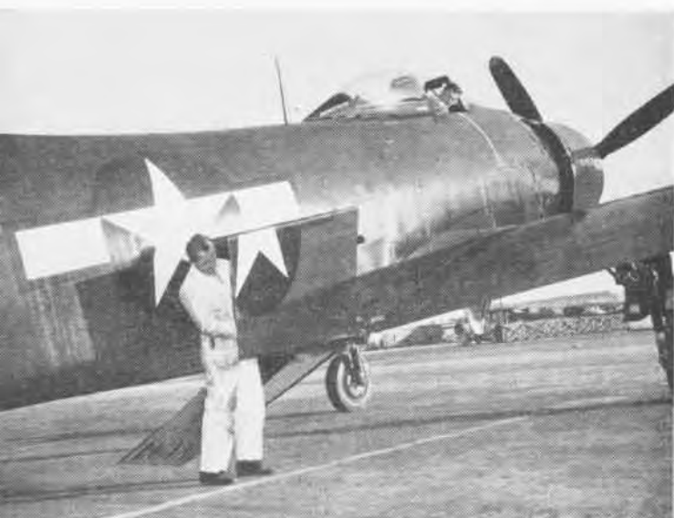
SKYRAIDER'S DIVE BRAKES ARE HUGE FLAPS HINGED FROM FUSELAGE
