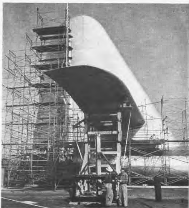
RED BEACON ON SCAFFOLD PROTECTS 80' TAIL FROM AIRCRAFT
