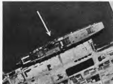
ISLAND WAS PARTLY COMPLETED IN 1942
