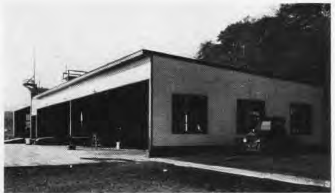
GLENVIEW RESERVE UNIT HAD FINE HANGAR, GROUND TRANSPORT
