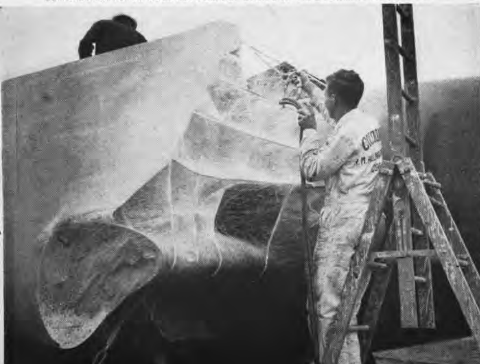
COMPOUND SPRAYED OVER NETWORK OF STRIPS OF TAPE FORMS A CLINGING COBWEB FILM
