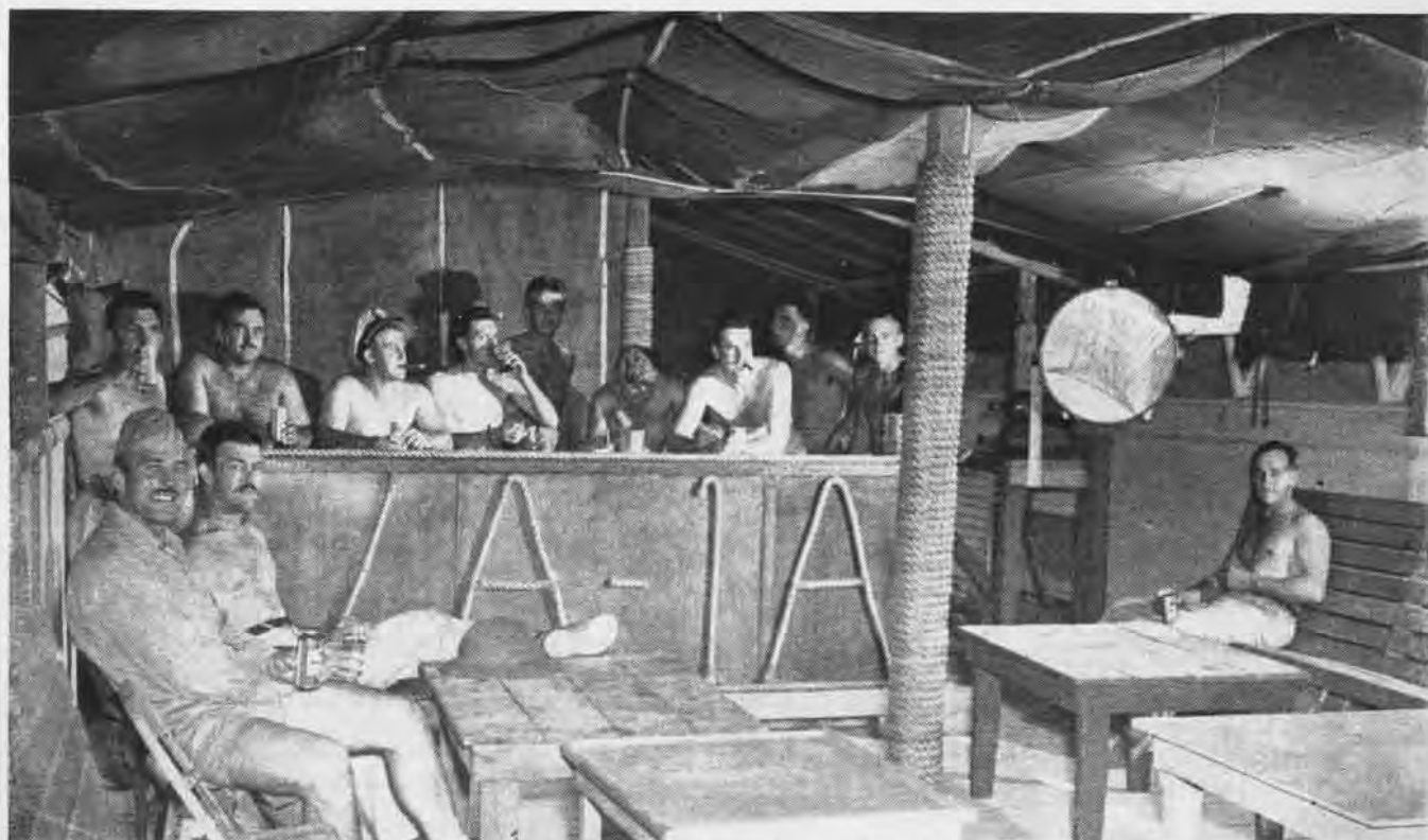
EXCLUSIVE ROPE ROOM WAS BUILT BY OFFICERS OF VA-1A FROM JUNKED MATERIAL; ELECTRICAL GENIUS MADE AN ICE MACHINE
