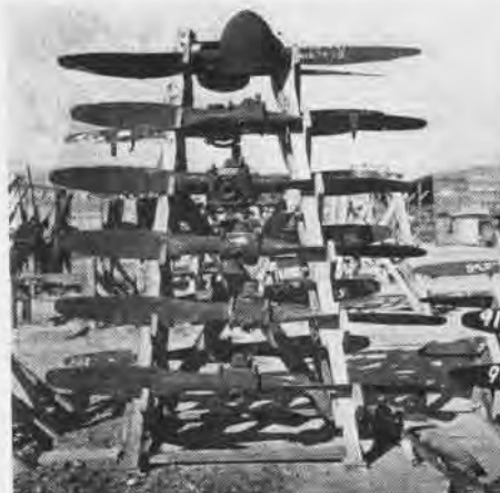
NEW PROPELLER RACKS DEvised AT ALAMEDA CONSOLIDATE STORAGE AREAS, SAVE SPACE
