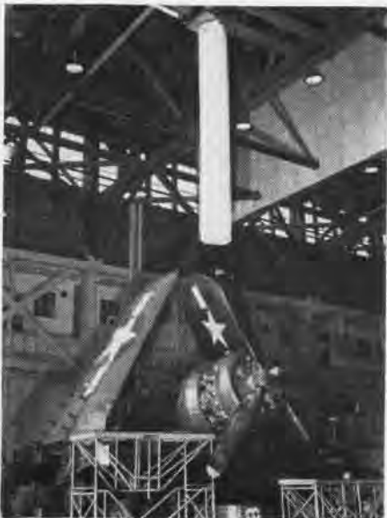
SLEEVES CONVEY HEAT TO WORKING AREA
