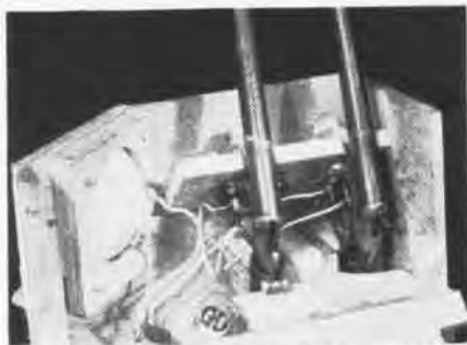
SAFETY OFFICER CUTS NIGHT FLYING HAZARDS
