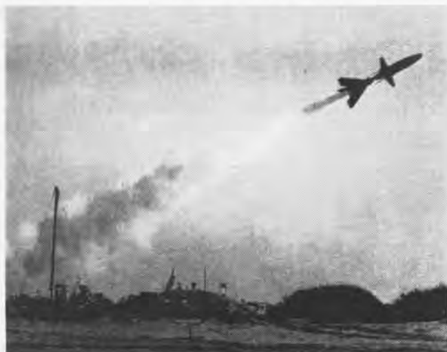
The NACA Tiamat flies a controlled predetermined track and is tracked by radar while data are telemetered back to ground
