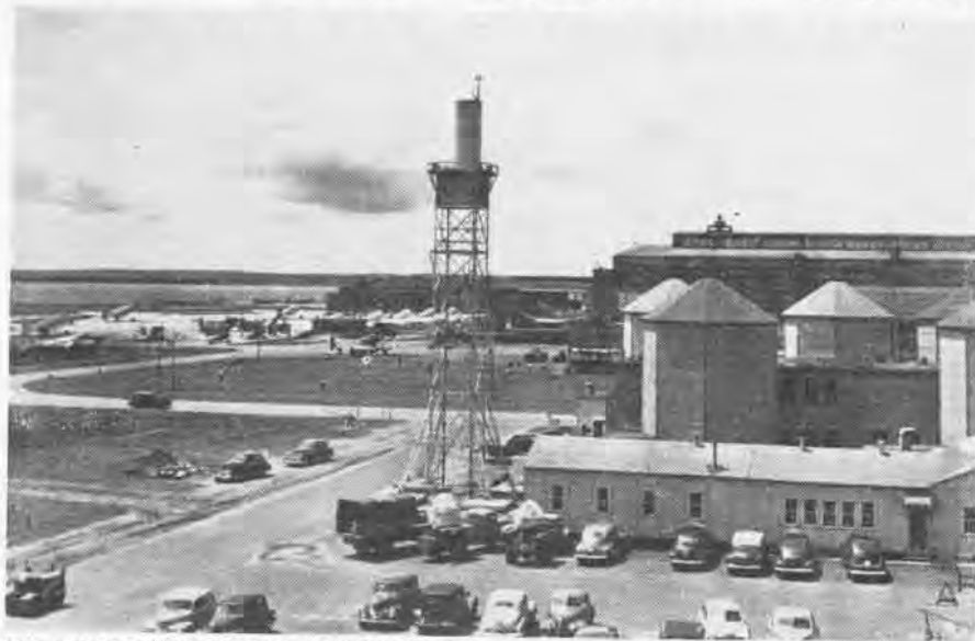
THE HEIGHT FINDER ANTENNA IS MOUNTED ON A 67-FT. TOWER TO ELIMINATE GROUND CLUTTER
