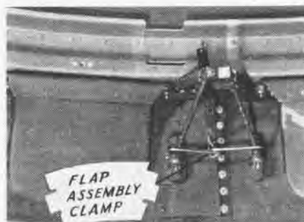
SIMPLE CLAMP HOLDS SB2C'S FLAP ASSEMBLY
