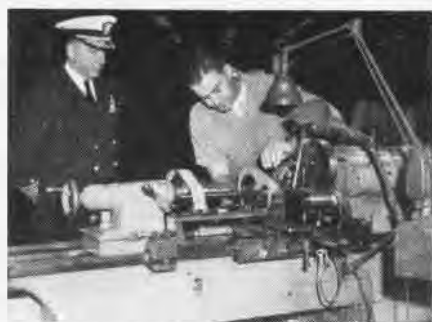
ADM. BLANDY WATCHES WORKER WIRE RESISTOR
