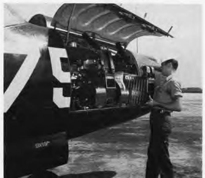
LOADING AMMUNITION ABOARD PHANTOM OR BANSHEE IS SIMPLE TASK
