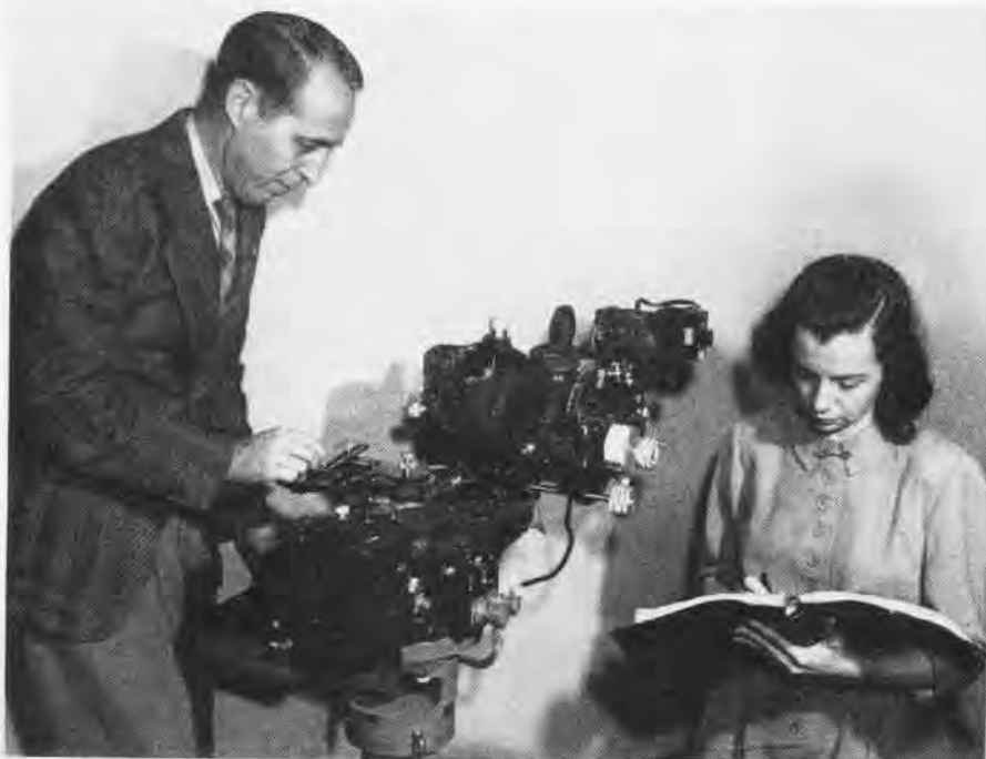
WORKERS CHECK NORDEN BOMBSIGHT COMPUTER; SIGHT WAS ONE OF PLANT'S WAR PRODUCTS
