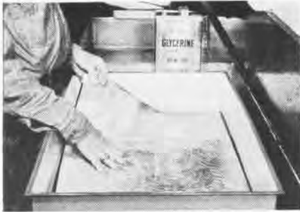
1 Prints are soaked in glycerin before being mounted to backing
