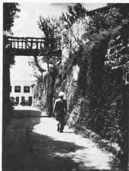
Lt. Cdr. Pomfrey inspects road cut through coral hill in middle of city
