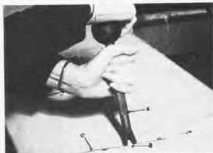
TOOL SPEEDS INSTALLATION OF FABRIC WIRE
