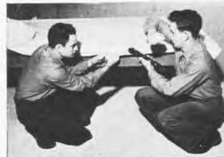
4 Aircraft fabric is stretched onto aluminum top table, stapled
