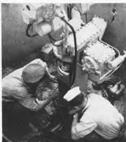
Crewmen check gun director electrical connection before putting it in service
