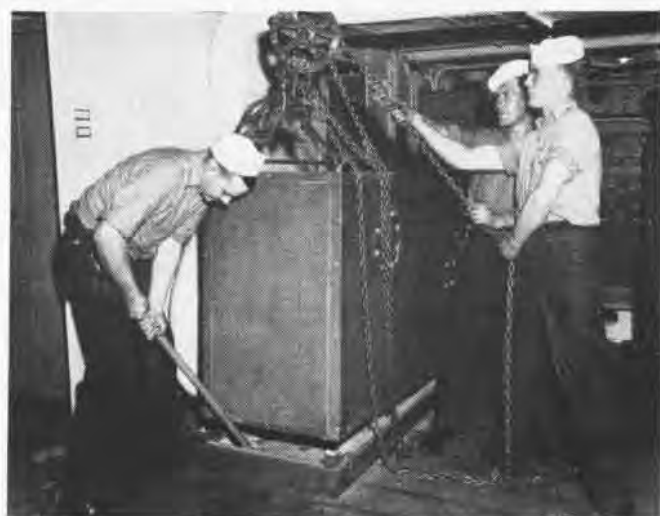
Removing dehumidification machine requires services of P. J. Cyr, SMIC, Z. A. Palmer, SA, G. W. Miles, SM, on Cabot
