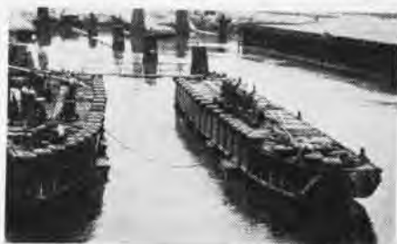
FLARED ENTRANCE TO SLIP WITH TIRE GUARDS
