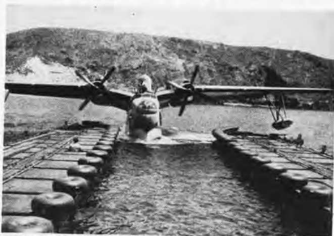
MARINER ENTERS SLIP; NOTE HOW WATER JET FORCES PLANE TO CENTER
