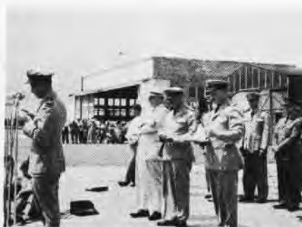
COMMISSIONING OF THE AVU(A) AT CHARLESTON
