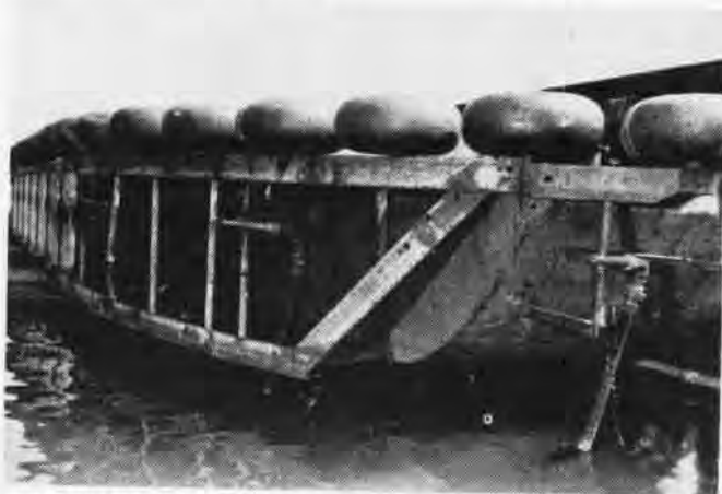
THREE WATER JET NOZZLES VISIBLE WHEN SLIP RIDES HIGH IN WATER
