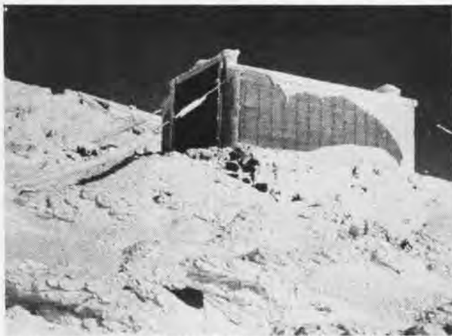
FOOT-THICK ICE COATS CABLES HOLDING HANGAR ON WIND-SWEPT PEAK
