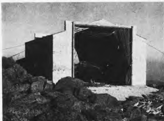
ANCHORED TO ROCKS BY CABLE, HANGAR PROTECTS PHANTOM TEST PLANE
