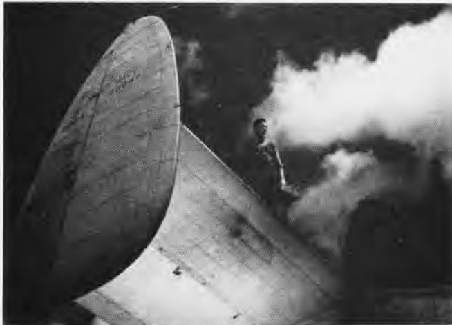
IN ROUGH WATER OPERATIONS THE RUDDER OFTEN HAD TO BE REPAIRED
