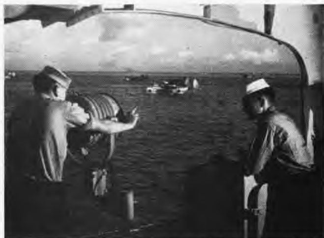
BLINKER IS USED AT THE BUOY FOR SHIP TO PLANE COMMUNICATIONS
