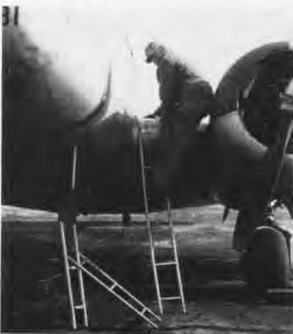
COLLAPSIBLE LADDERS BUILT AT CHERRY POINT
