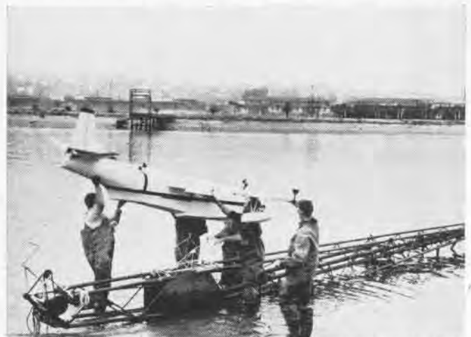
MOVIE CAMERA RECORDS CATAPULTING OF A MOTORLESS FLYING MODEL
