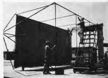
CHUTE LOFT EASILY PORTABLE TO FIELD SITE
