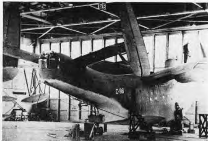
LIQUID ROCKET JATO WAS TESTED INSTALLED AFT OF PBM TUNNEL HATCH
