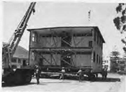
SECTION OF BARRACKS MOVES DOWN THE STREET
