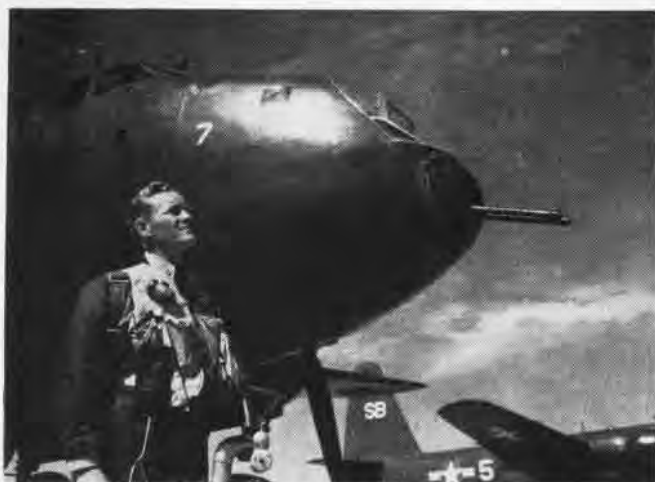
P2V-1 NEPTUNE HAD A NOSE TURRET WITH TWIN .50 CAL. GUNS MOUNTED
