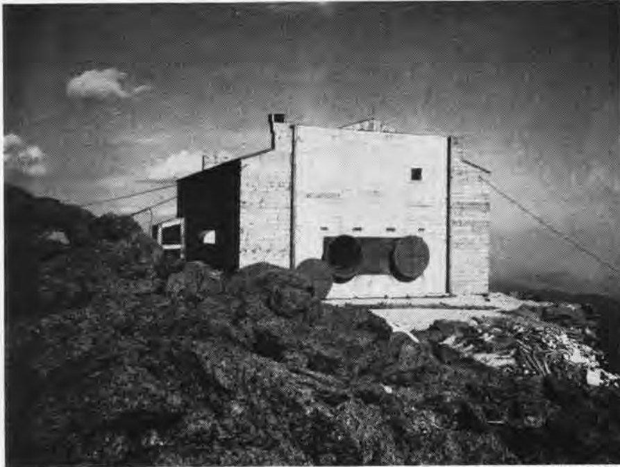
BUTLER BUILDING ON MT. WASHINGTON'S SUMMIT SHOWING JET AIR INTAKES AND ROCKY TERRAIN
