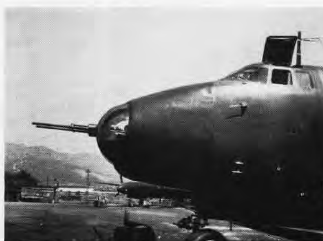
NEPTUNE NOSE ARMAMENT FEATURES TWIN 20 MM. CANNON IN TURRET
