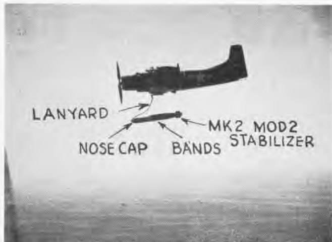
TORPEDO DROPS AWAY AFTER THE DOUGLAS BOMB EJECTOR RELEASES IT
