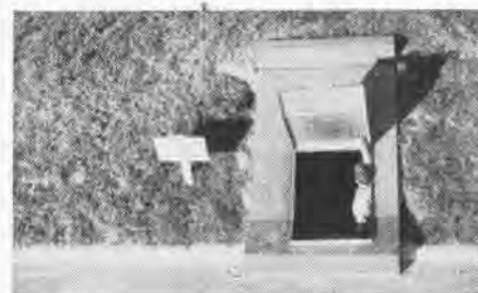
STORAGE COVERS IN USE AT NAS NEW ORLEANS
