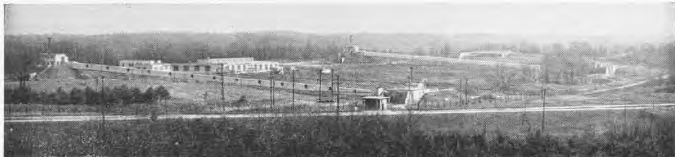
ONE OF TWO AREAS DEVOTED TO HANDLING AND POURING OF CAST EXPLOSIVES; DEPOT SITE WAS CHOSEN FOR REMOTENESS FROM POPULATION CENTERS
