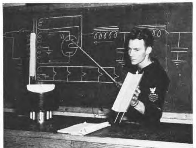
J. B. CONYERS, ATI, EXPLAINS RECTIFIER TUBE BY USE OF MOCKUP
