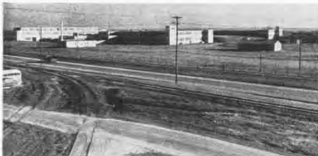
AREA AROUND PYROTECHNICS PLANT BRISTLES WITH LIGHTNING ARRESTERS
