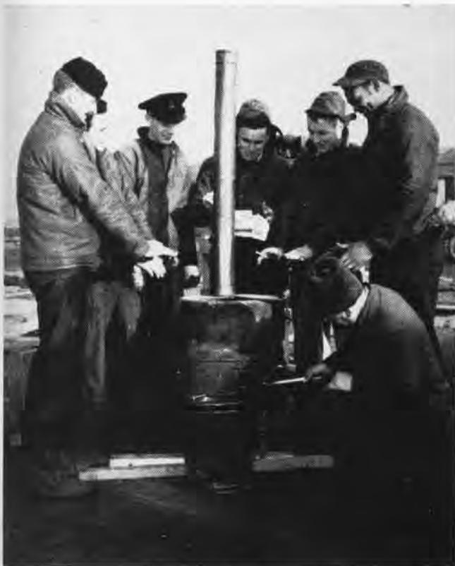
Groundcrewmembers of VR-6 thaw out around an open-air stove between engine checks before the ready room hut was built
