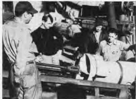
MORRIS DAM TORPEDO TEST WORKERS LOAD TUBE
