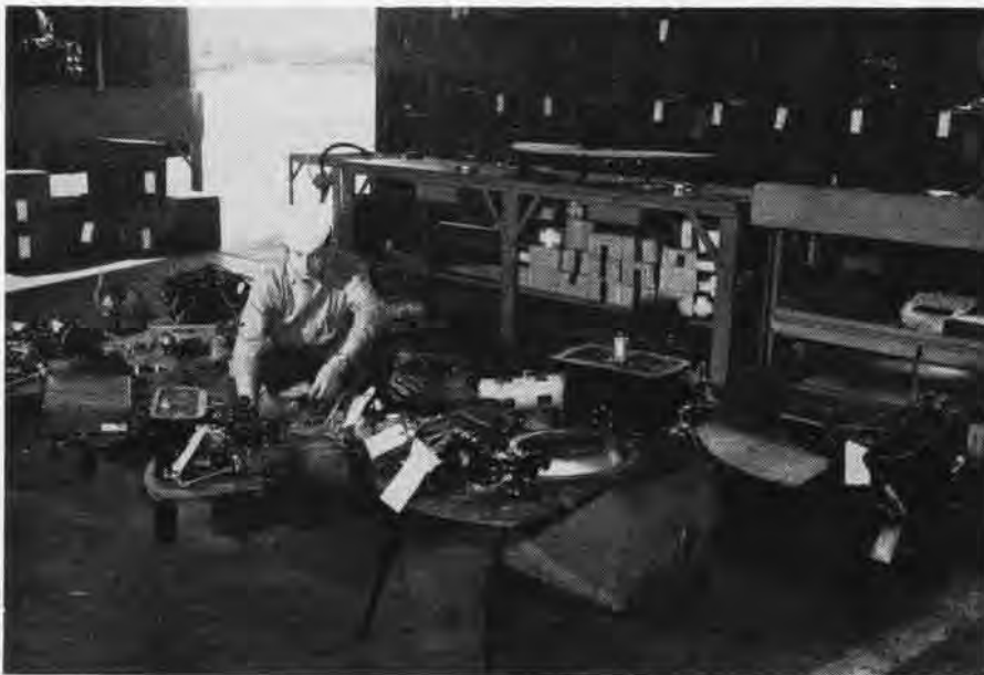
MACHINIST'S MATE PREPARES ACCESSORY BOARD FOR LATER MOUNTING OVER THE ENGINE SHAFT
