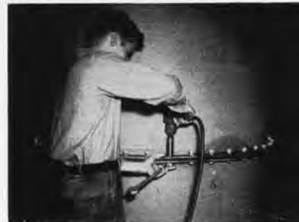
BOLTED AND SEALED FOR FINAL LEAKAGE TESTS
