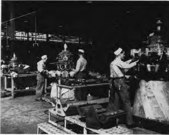
DISASSEMBLY OF ENGINE FOR INSPECTION AND PROCESSING COMES FIRST
