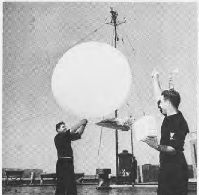
RADIO-SONDE TRANSMITTERS SOUND UPPER ATMOSPHERE ECONOMICALLY leased by universities, laboratories and commercial airlines.
