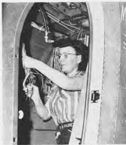
WOMAN ELECTRICIAN INSTALLS WIRING IN SNB-4
