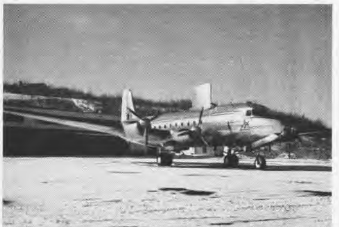
TO PROBE AIRCRAFT ICING, SHARK-LIKE FIN IS PUT ON NORTH STAR
