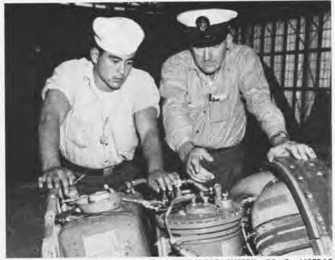
CHIEF GORWOOD EXPLAINS F4U-4 HYDRAULIC SYSTEM TO E. LIPTRAP
