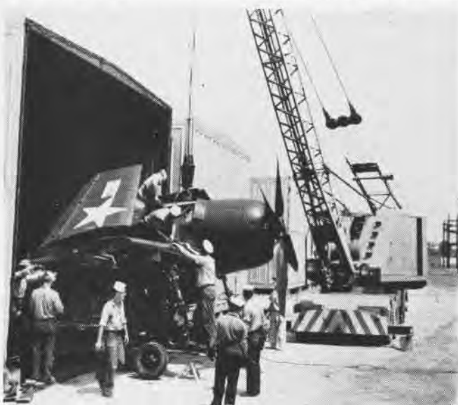
PLANE IS HOISTED OFF TRACK PREPARATORY TO MINOR ASSEMBLY WORK
