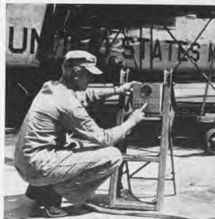
MAGNETO TESTER ISOLATES BALKY CYLINDERS
