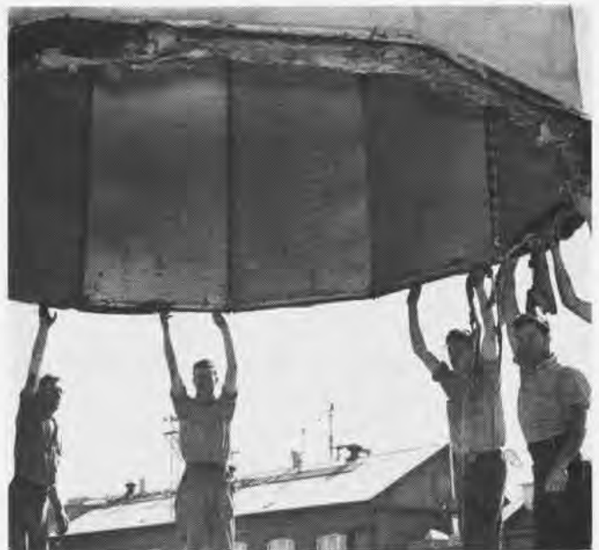
REACTIVATION CREW GUIDES PRESERVATIVE COVER AS IT IS HOISTED
