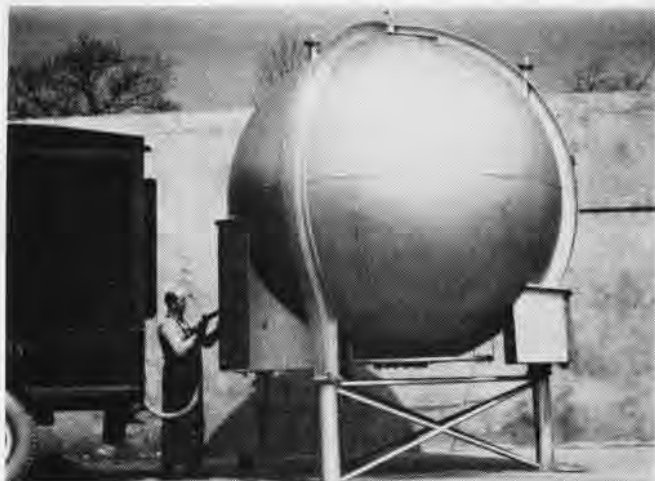
ONE TYPE of liquid oxygen storage at Lake Denmark is this spherical tank; fluid is transferred by hose from truck to tank
