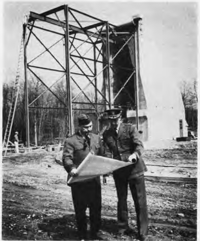
NEW TEST stand for higher power rocket engines nears completion; Ex-C.O. Capt. Jackson and Cdr. Seiler, former Exec, study plans
