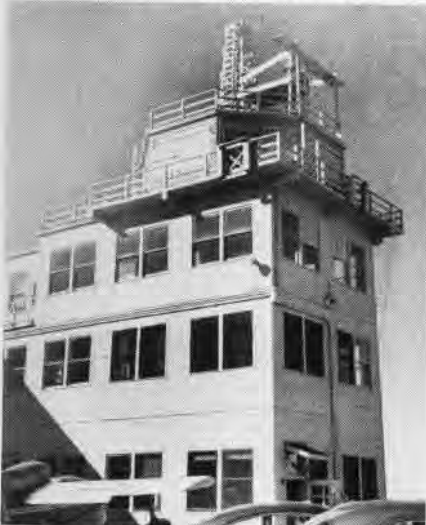
BOARDED WINDOWS, CURTAINS IN EX-TOWER
