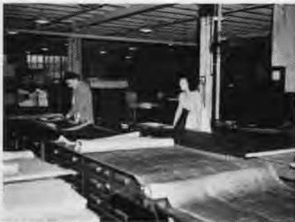
DATA IS INSPECTED FOR LEGIBILITY AT TRD
