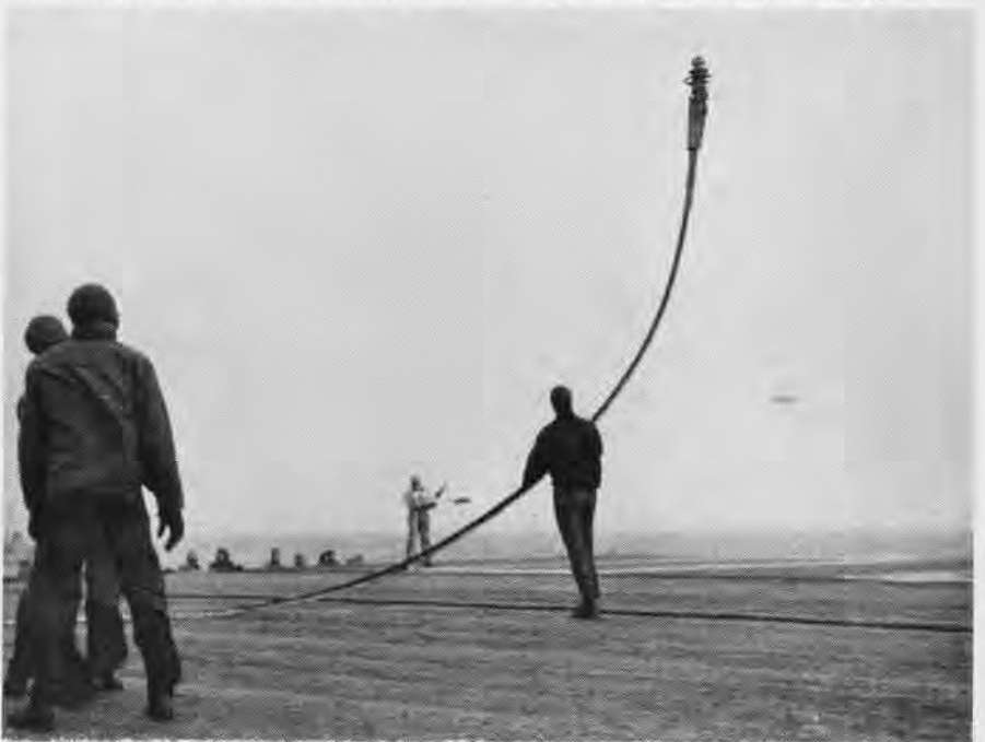
HINDU ROPE trick? When ZP-1 was operating off the CVE Mindoro off the Virginia capes, refueling the airships while in flight was practiced. In this picture, the fueling hose is in the process of being hoisted up to the blimp so that fuel can be pumped to its tanks.
